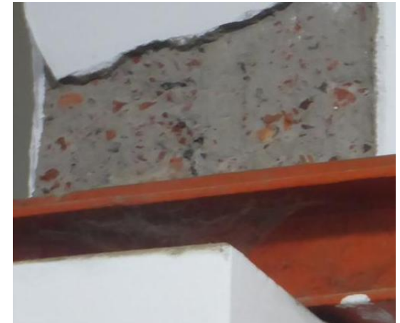
Brick Aggregate Observed
