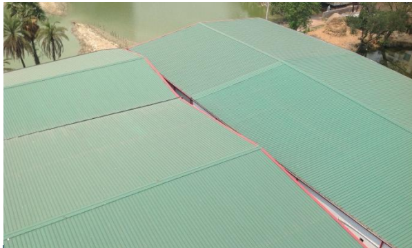
View of Sheds from Main Building Roof
