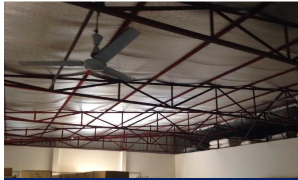
Lightweight Steel Roof to Ground Floor Shed 1
