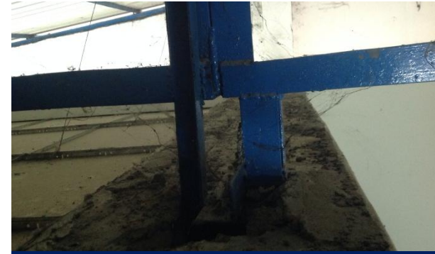
Truss to Column Connection Detail
