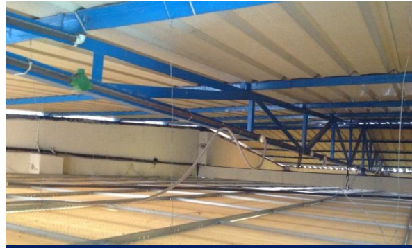
Steel Trusses to Dining Area Roof
