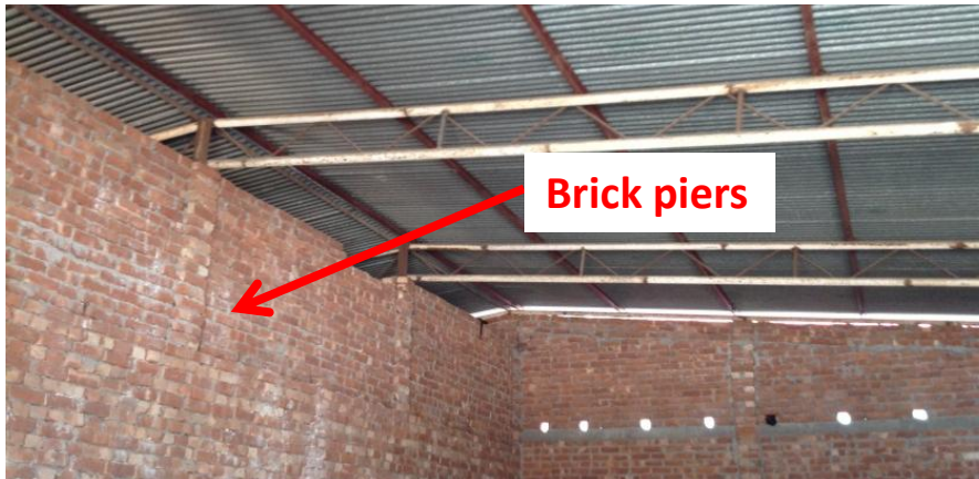
Steelwork supported on smaller brick piers
