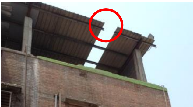
Cut roof purlin
