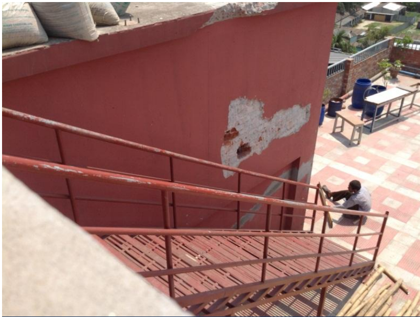
Water tank slab alteration
