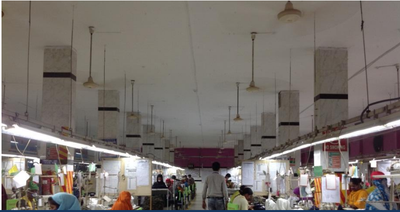
Flat slab at Level 3 Ceiling
