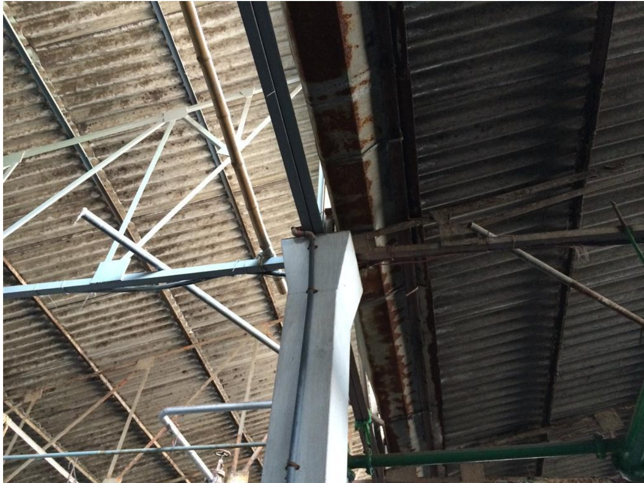
Roof connections – Dyeing shed
