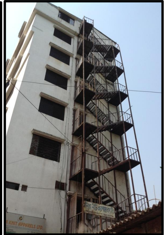
External Fire Stair
