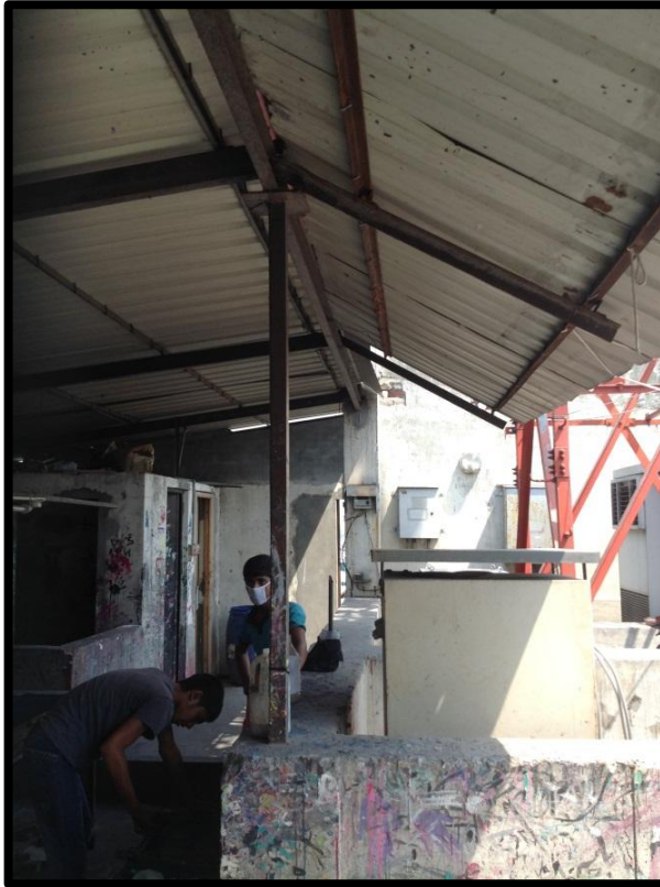
Building Steel Roof
