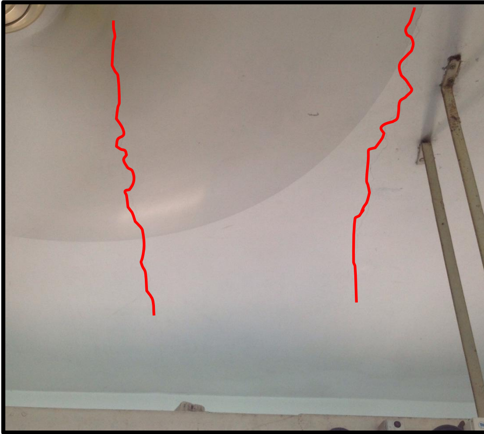
Flexural Cracking in Floor Slab Soffits
