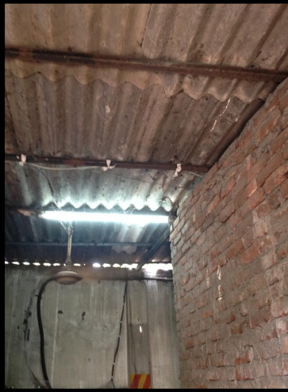
Generator Room Steel Roof
