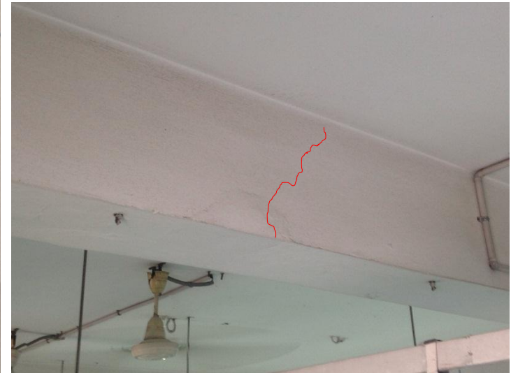
Beam Cracking
