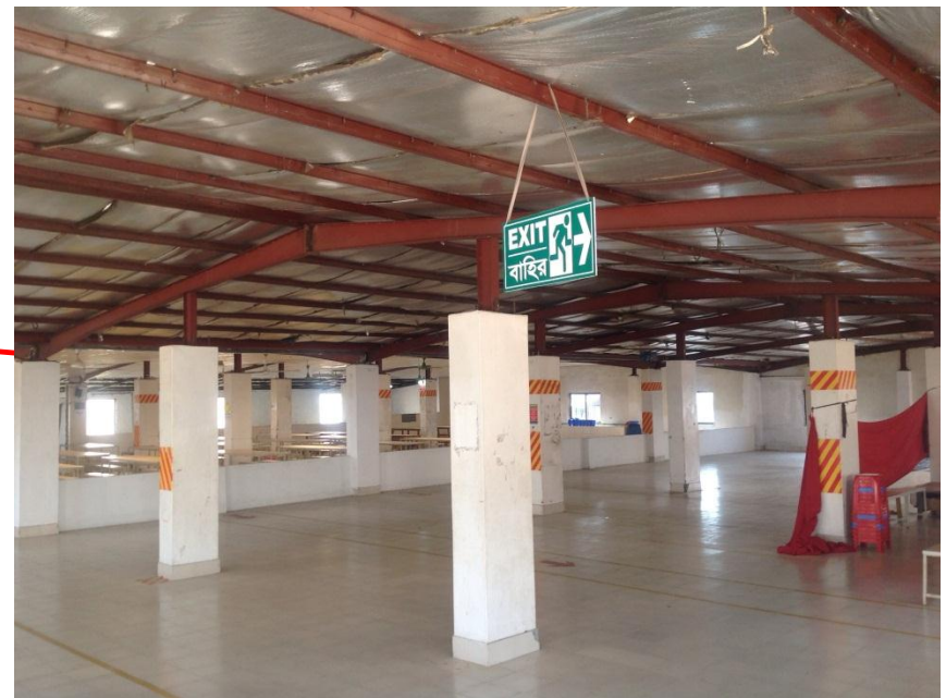
Roof structure to Dining Area
