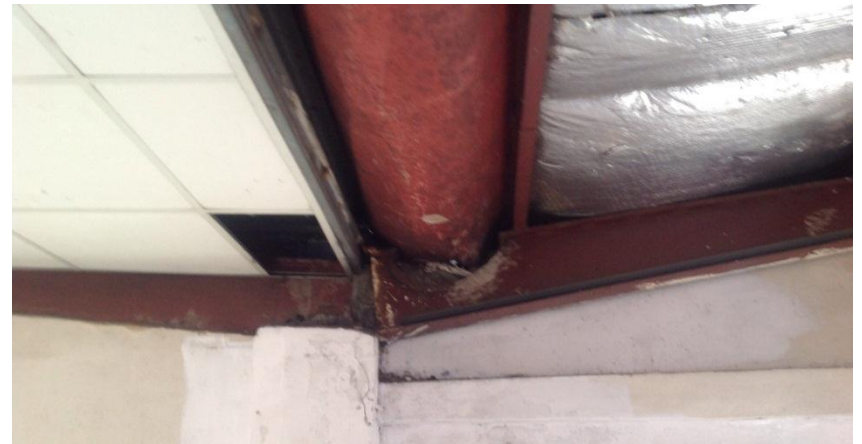
Steel Rafter – notched for gutter
