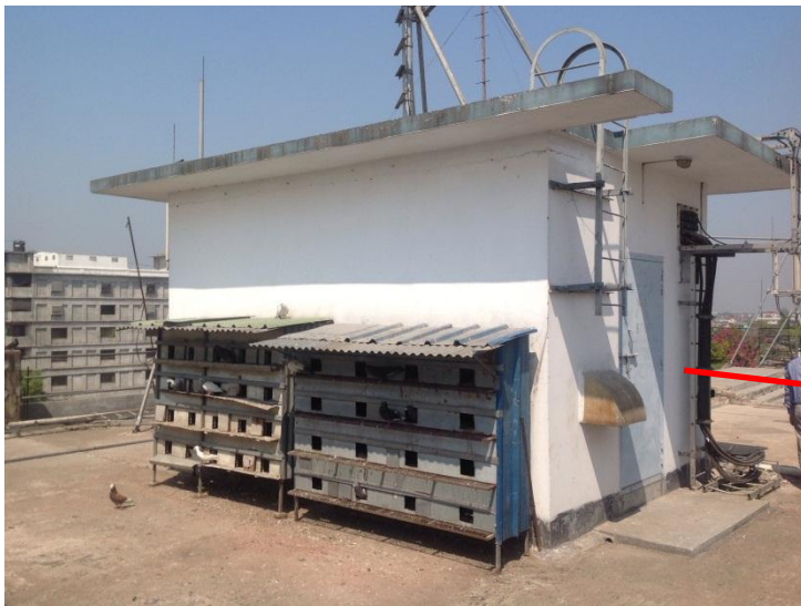
Roof Antenna House
