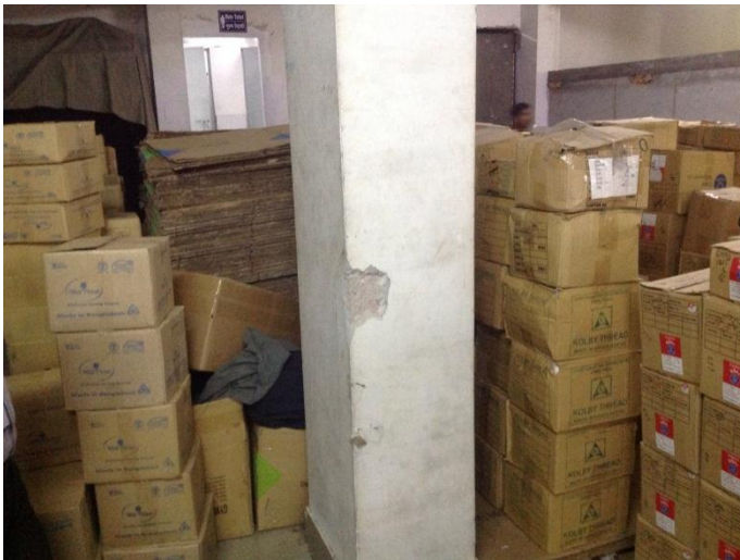
Tested Ground Floor Column – Brick Chips
