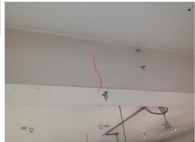
Beam Cracking
