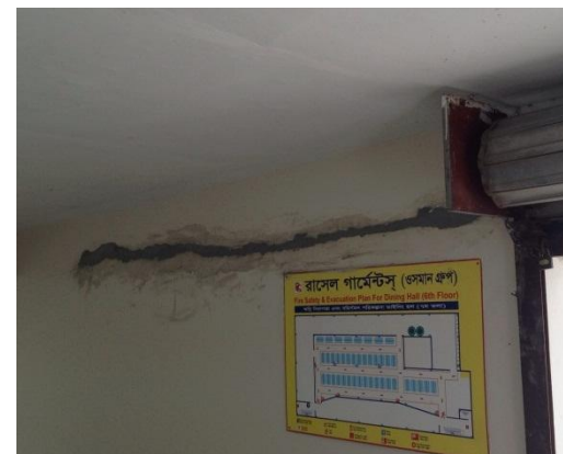
Filled Crack to 6 th Floor Wall
