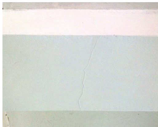
Filled Crack to 5 th Floor Beam
