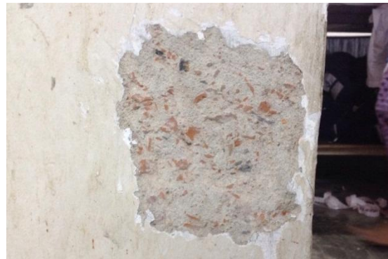
Tested Column - Bureau Veritas
