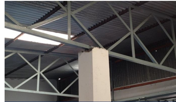
Truss to Column Connection Detail
