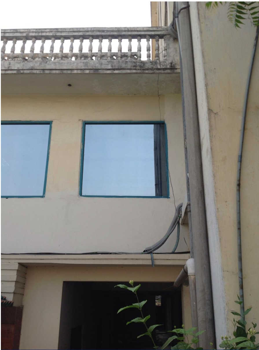
Junction between 4- and 7-Storey Buildings
