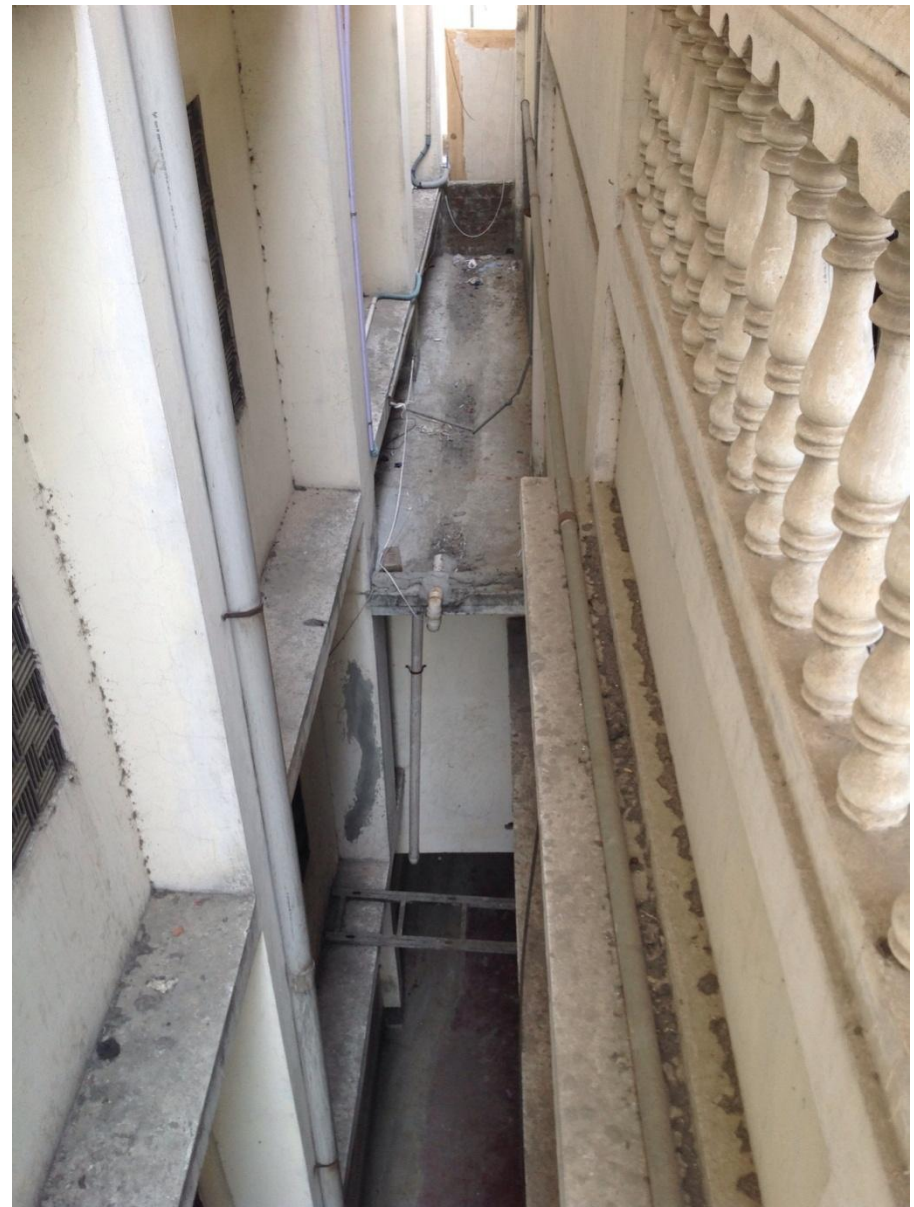
Junction between 4- and 7-Storey Buildings
