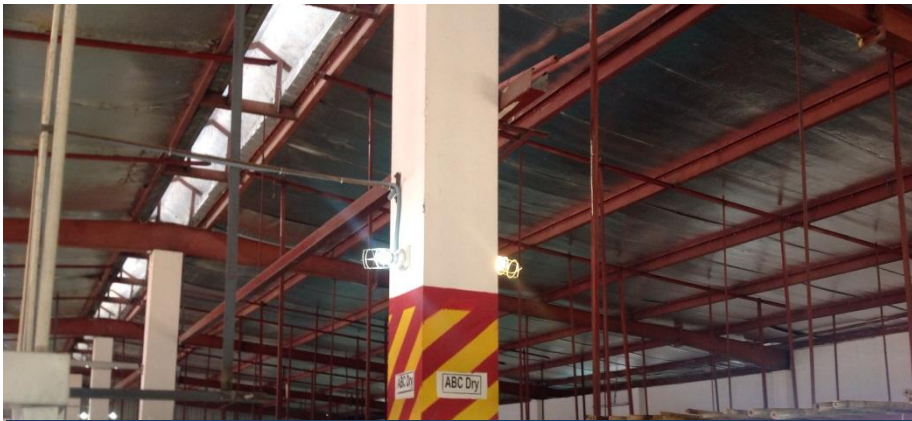
Printing Shed – no roof bracing
