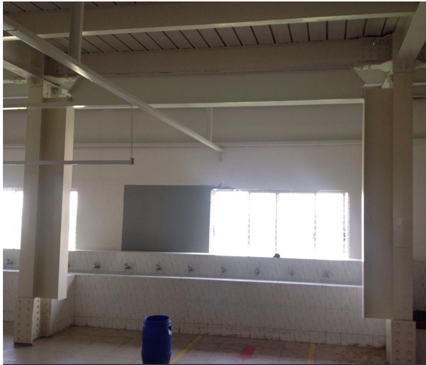
Typical portal brace – 3 rd to 5 th floors
