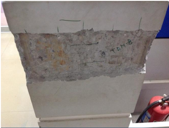
Stone aggregate in columns
