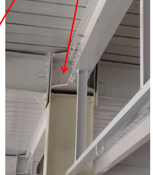
General lack of fit of connections in steel frame
