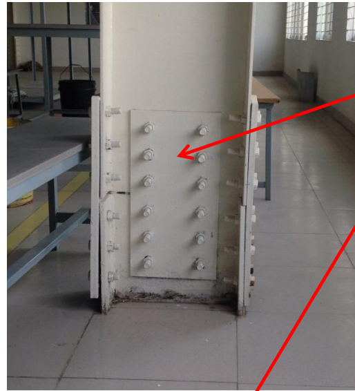
General lack of fit of connections in steel frame
