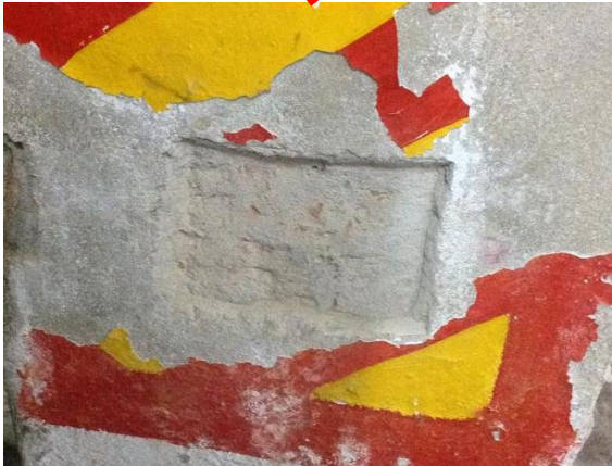
Phases I & II: Tested Ground Floor Column – Brick Chip Aggregate
