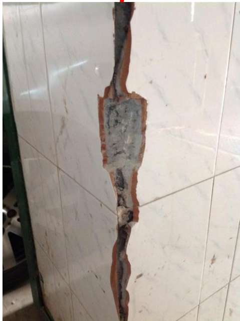
Phase III: Tested Ground Floor Column – Stone Aggregate
