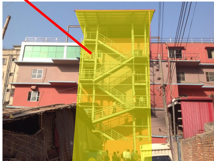
External steel stairs
