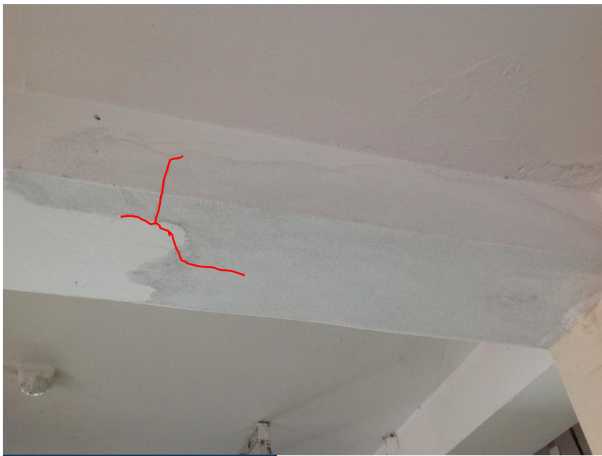
Beam cracking
