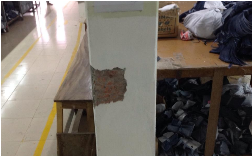
Tested Ground Floor Column – Brick aggregate
