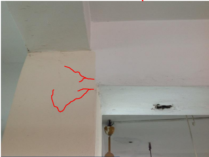
Column cracking
