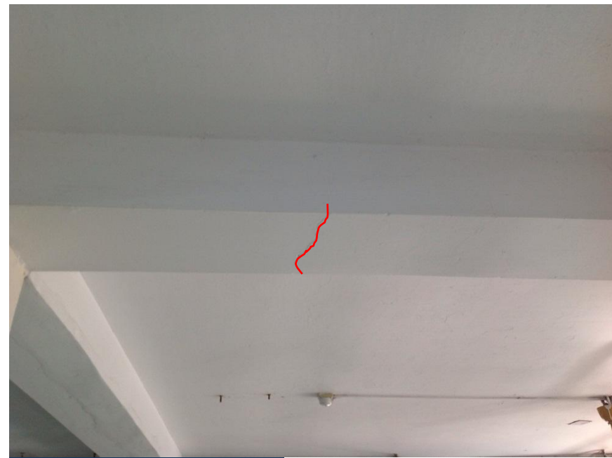
Beam cracking
