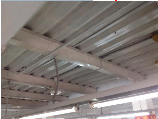
Stair ope in-filled
