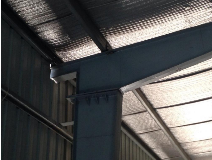
Column-to-Haunch Connection Detail
