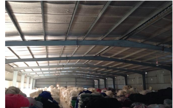
Bracing system missing from Raw Materials Godown Building
