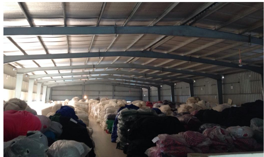
Yarn Storage to Raw Materials Godown Building
