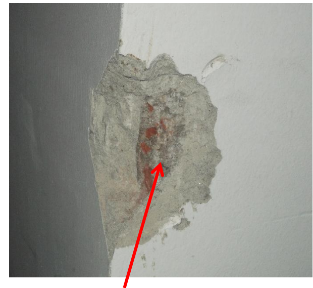
Checked Ground Floor Column – Brick Chips
