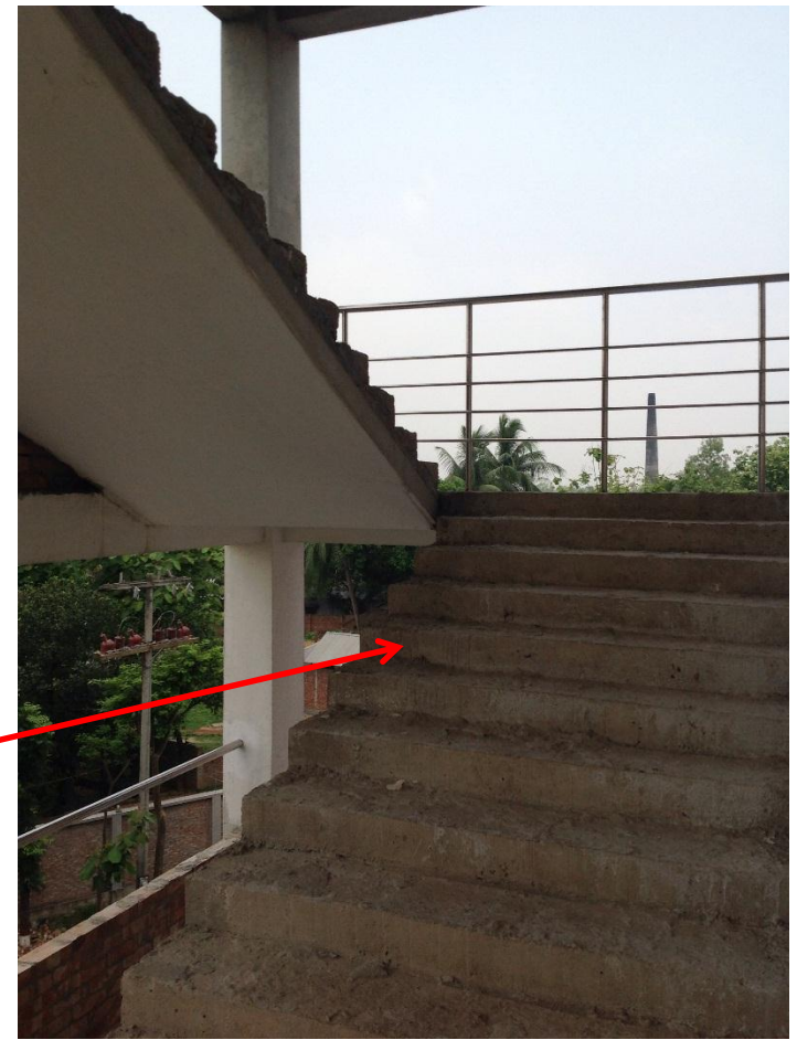
Stairs at south side of the building
