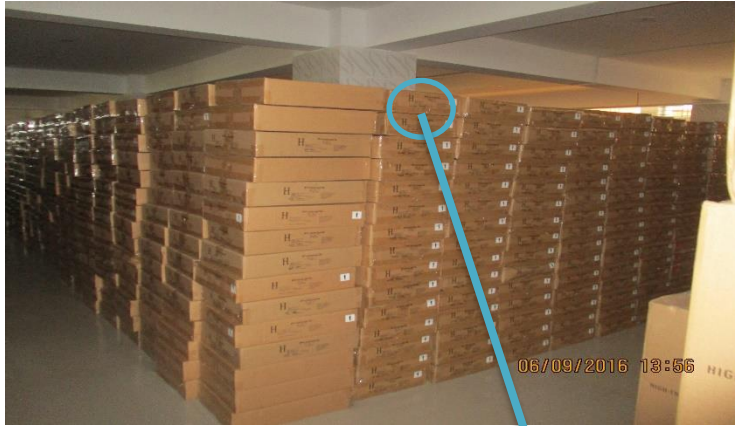
High Loading observed on 6 th Floor
