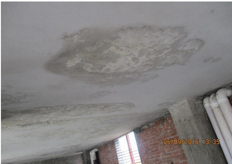
Dampness found on the bottom slab of RCC water Tank
