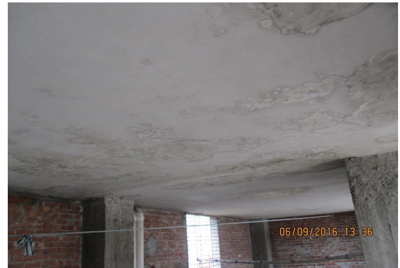
Dampness found on the bottom slab of RCC water Tank
