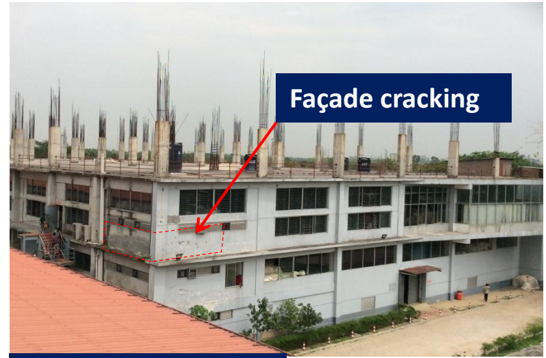
Façade cracking
