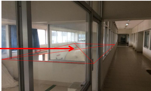
Mezzanine as constructed
