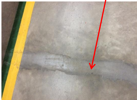
1 st floor slab
