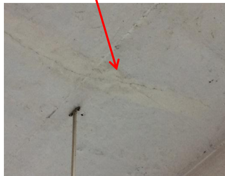
2 nd floor slab soffit
