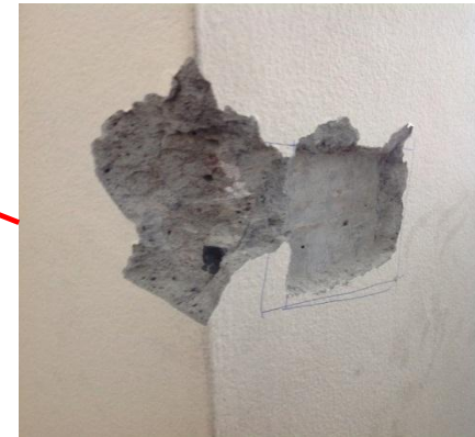
Column showing stone aggregate.
