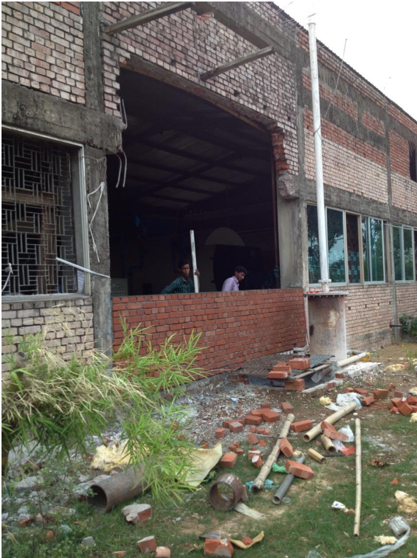
Opening without propping – Boiler building
