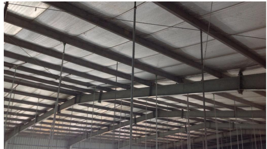
Only Horizontal Bracing provided to Main Building
