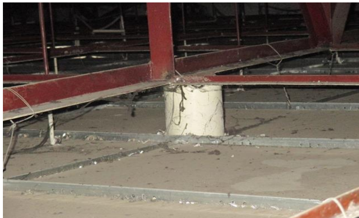
Steel pipe to truss connection for shed-2
