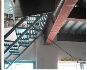
Steel stair at south poorly connected with I beam of deck slab
