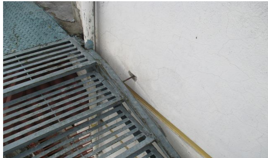
Apparently non-engineered steel stair poorly connected with north façade
