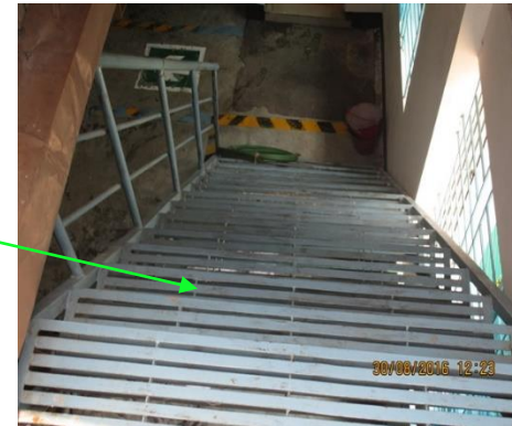
Steel stair at south poorly connected with I beam of deck slab
