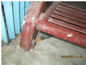
Steel stair poorly connected with partition wall and floor.
