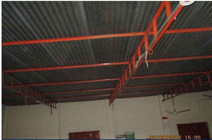
Steel truss are connected with brick column and periphery wall.
