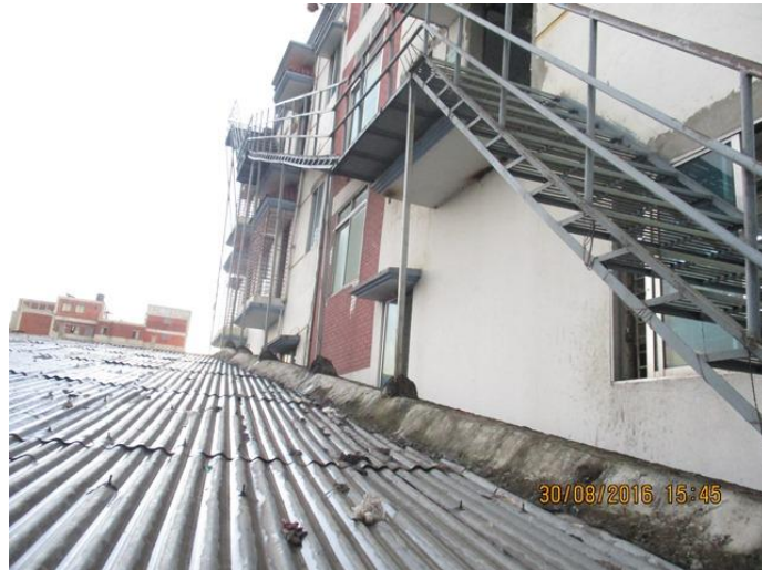
Apparently non-engineered steel stair poorly connected with north façade
