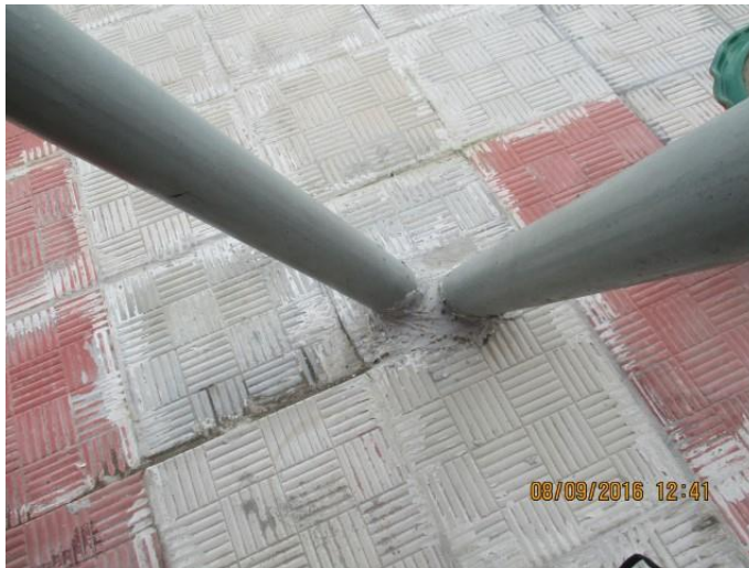
Branching column connection with slab
