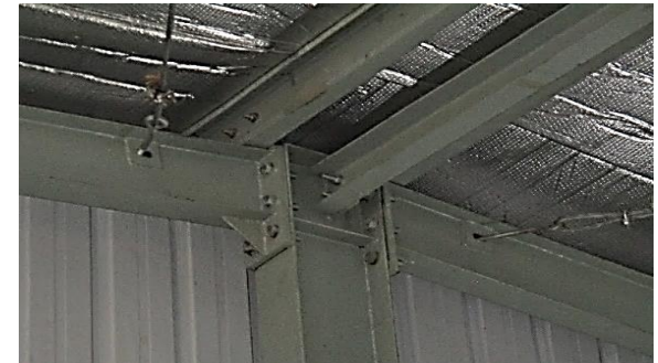
Typical connections of compression stud and bracing
