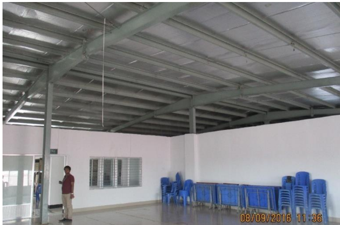
Roof top steel shed
