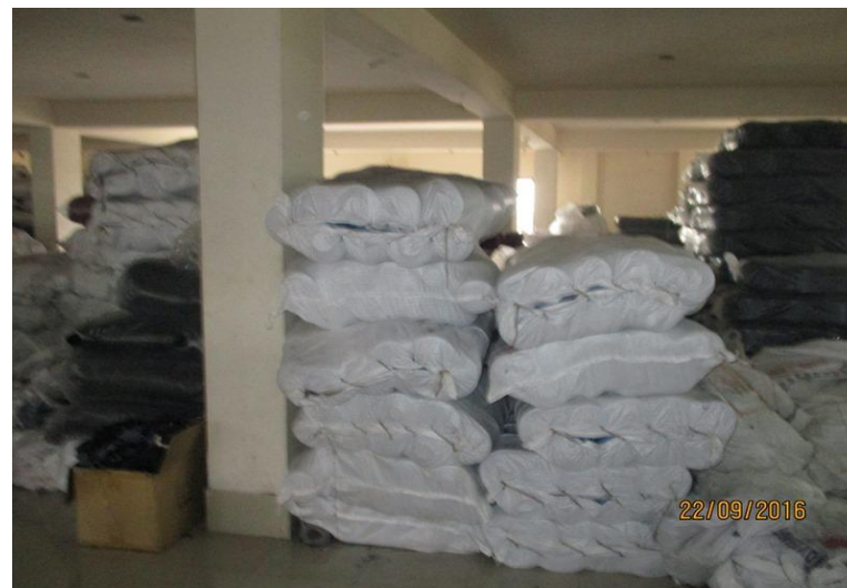
Over loaded area on 2 nd floor
