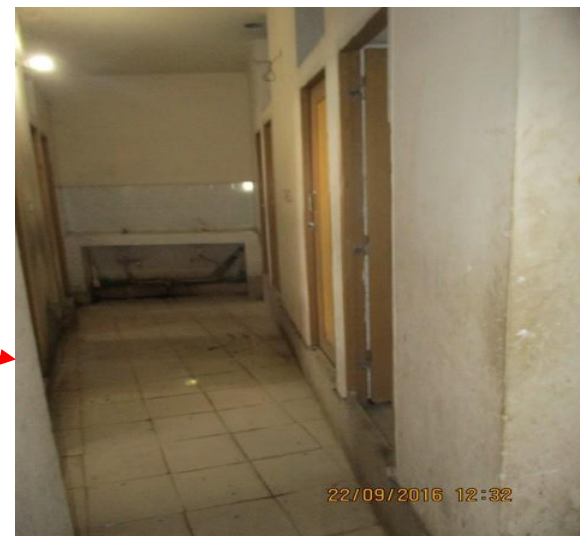
Toilet area on 3 rd floor
