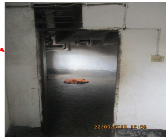
Mezzanine floor beside south stair case
