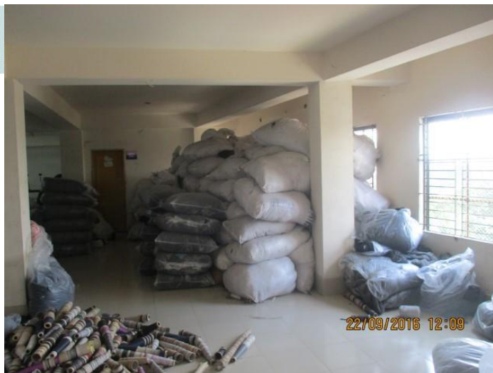
Over loaded area on 4 th floor
