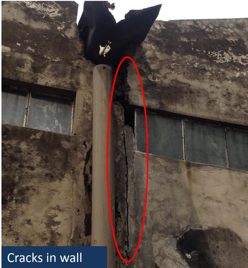
Location of beam cracking/wall movement
