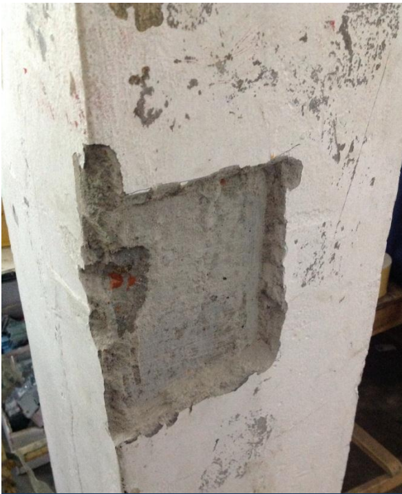
Brick aggregate in columns
