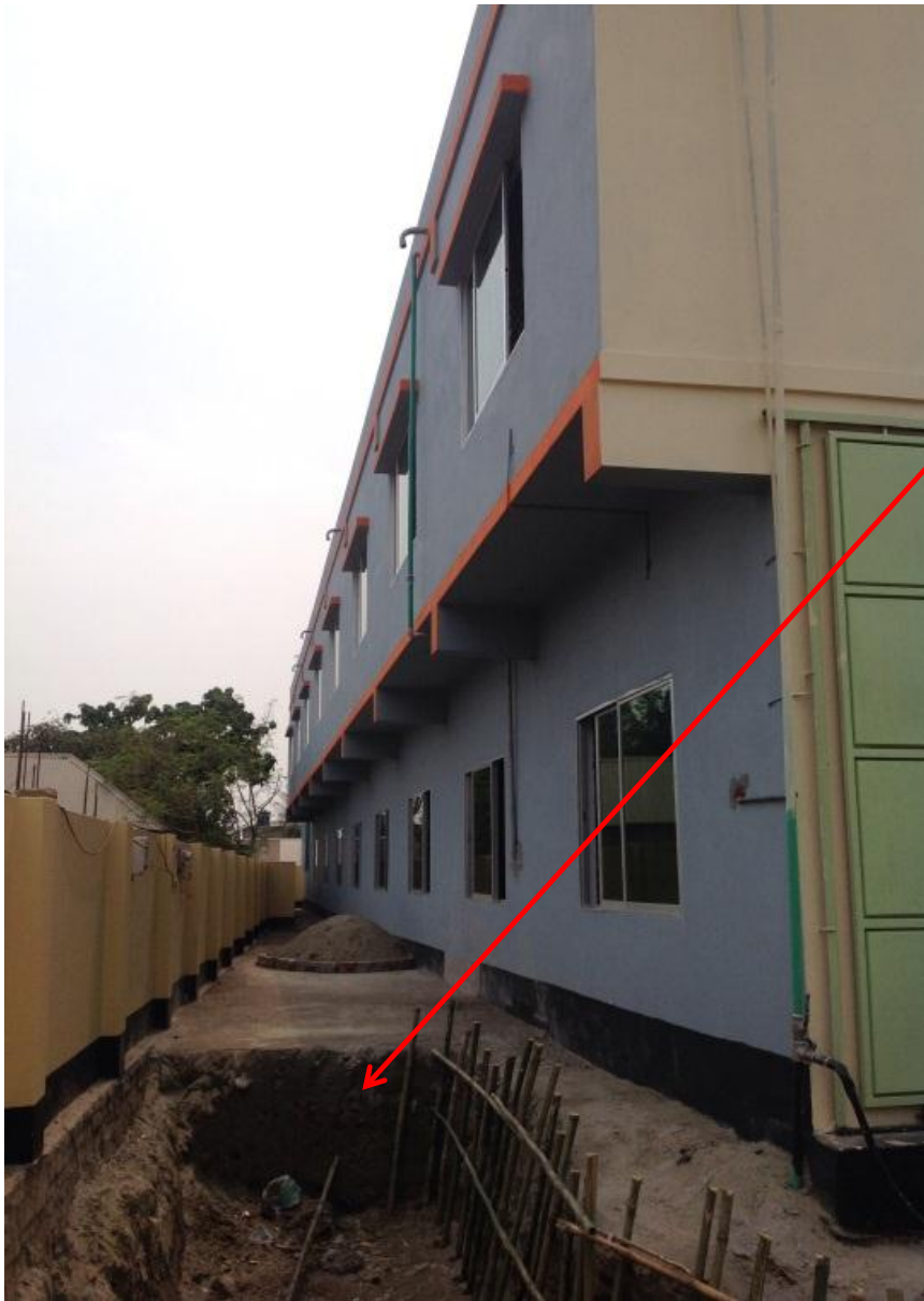
Open excavation near building
