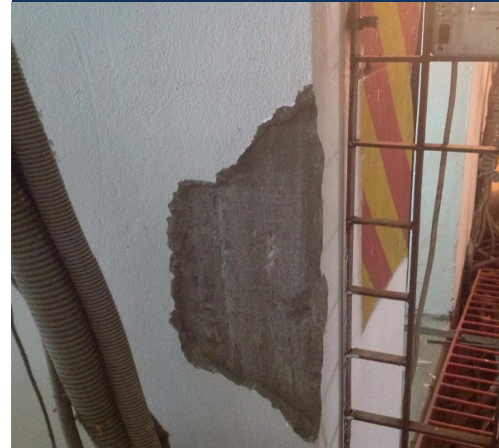
Tested Ground Floor Column
