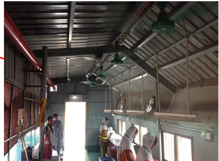
Lean-to structure on 6th Floor
