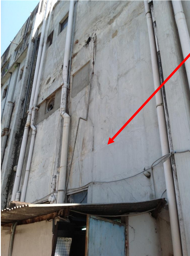
Cracks to building façade
