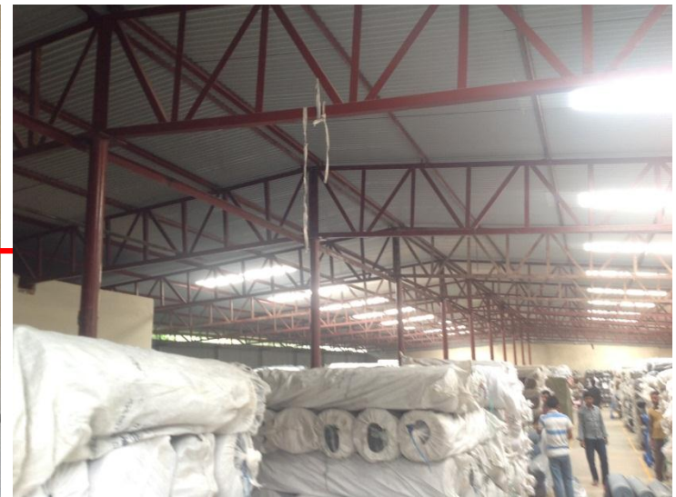
Additional steel structure
