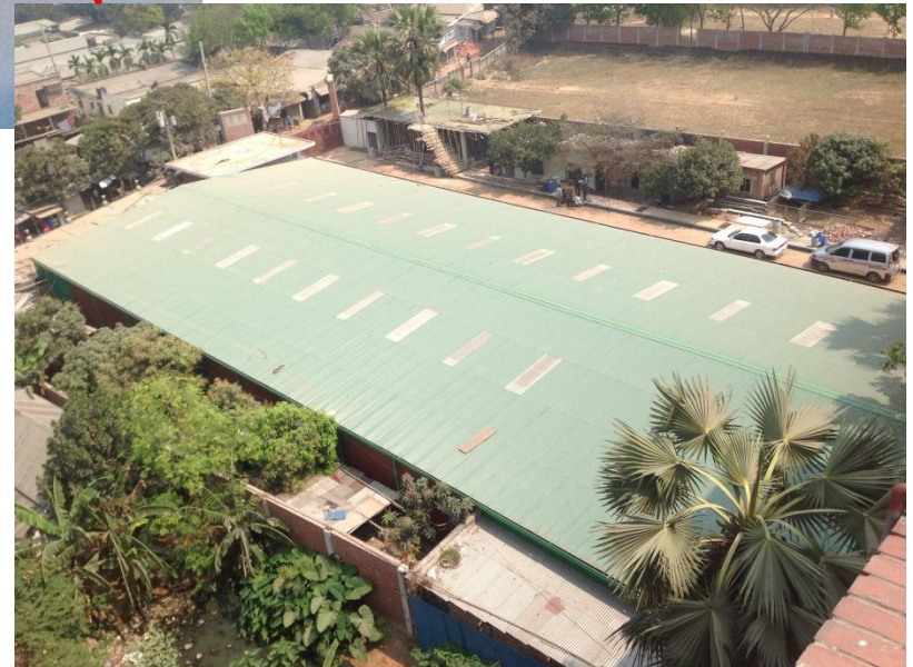
Additional steel structure
