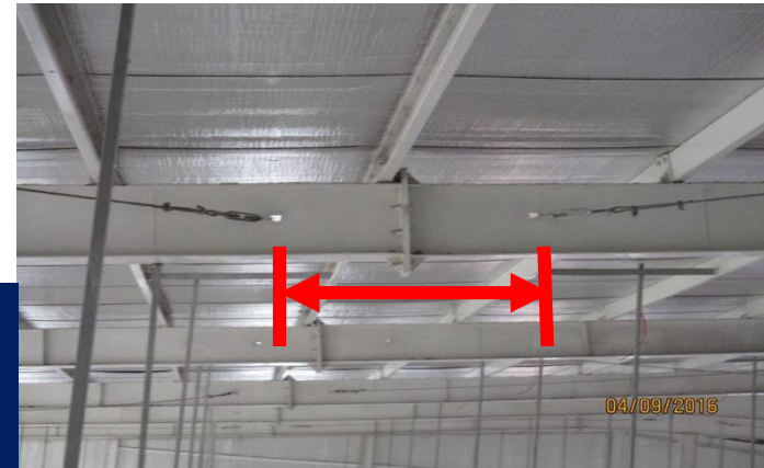
Plan bracing substantially away from vertical supports
