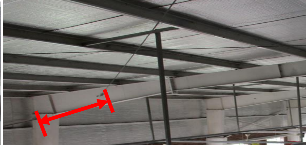
Plan bracing substantially away from vertical supports
