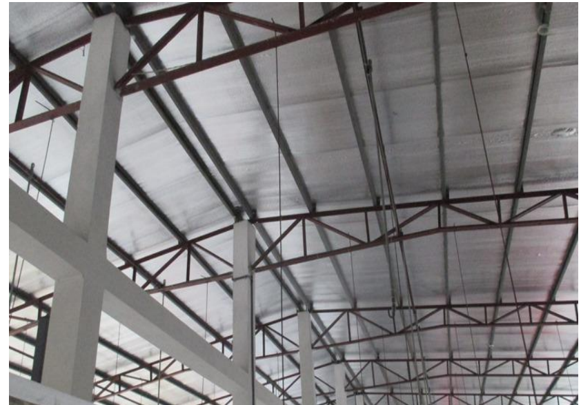
Roof at East
