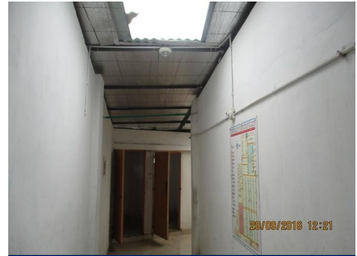
Toilet roof at East
