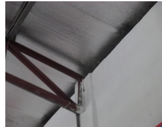
Truss section at East
