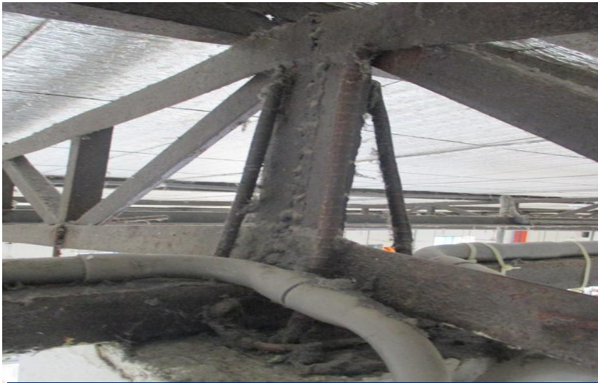
Truss connect with RC Column
