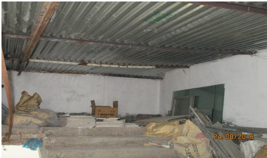
Stair case roof
