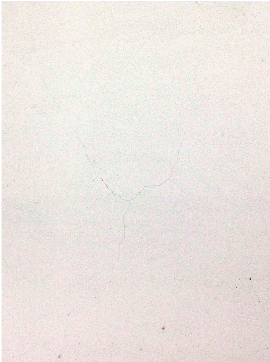
Cracking to underside of two-way spanning slab
