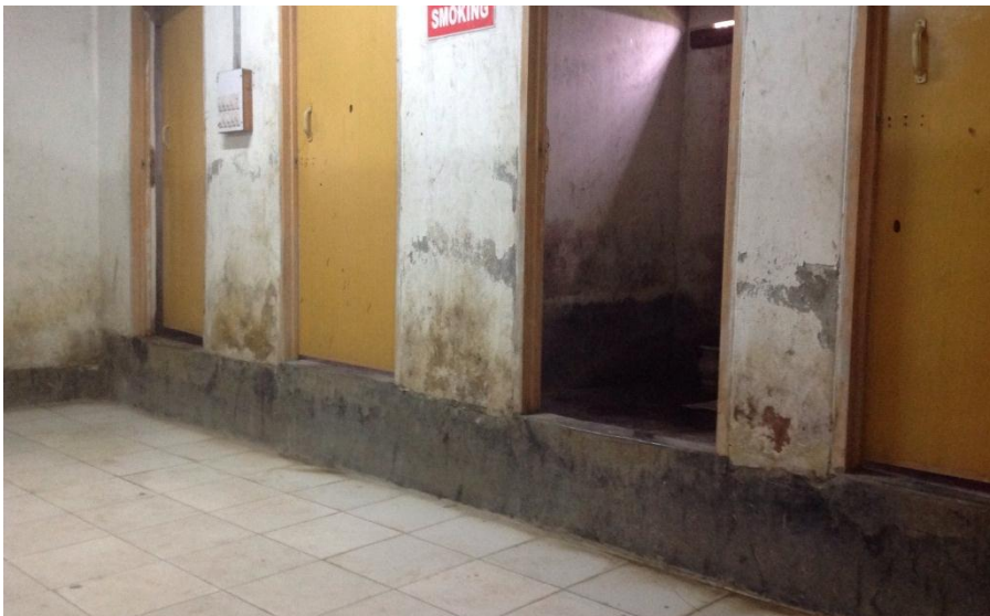
300mm Toilet plinth to 2 nd Floor
