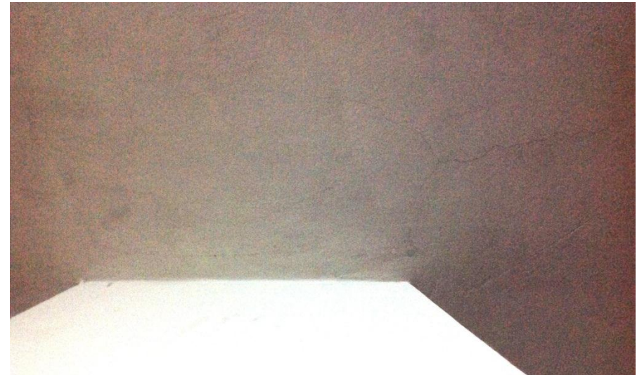
Cracking to underside of flat slab adjacent to column
