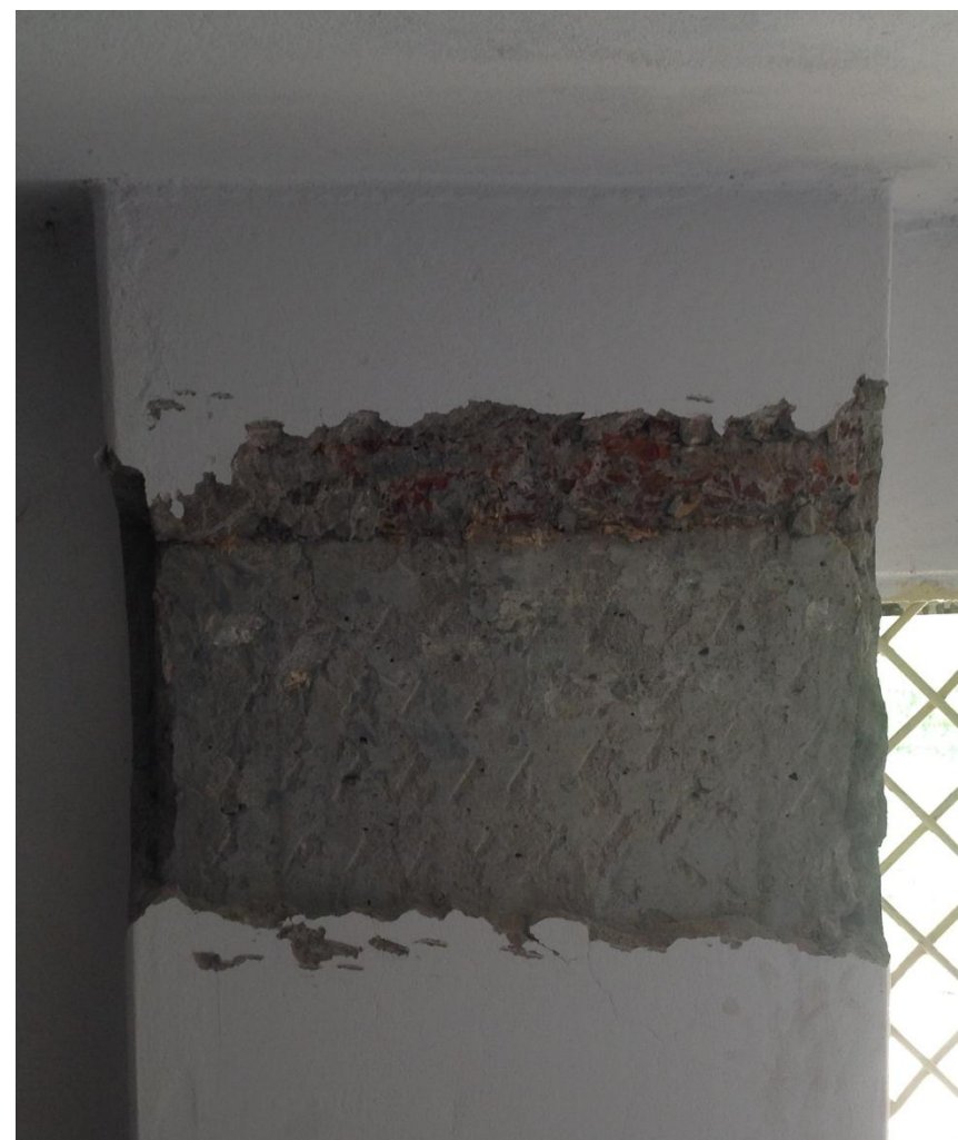
Exposed Column A/2
