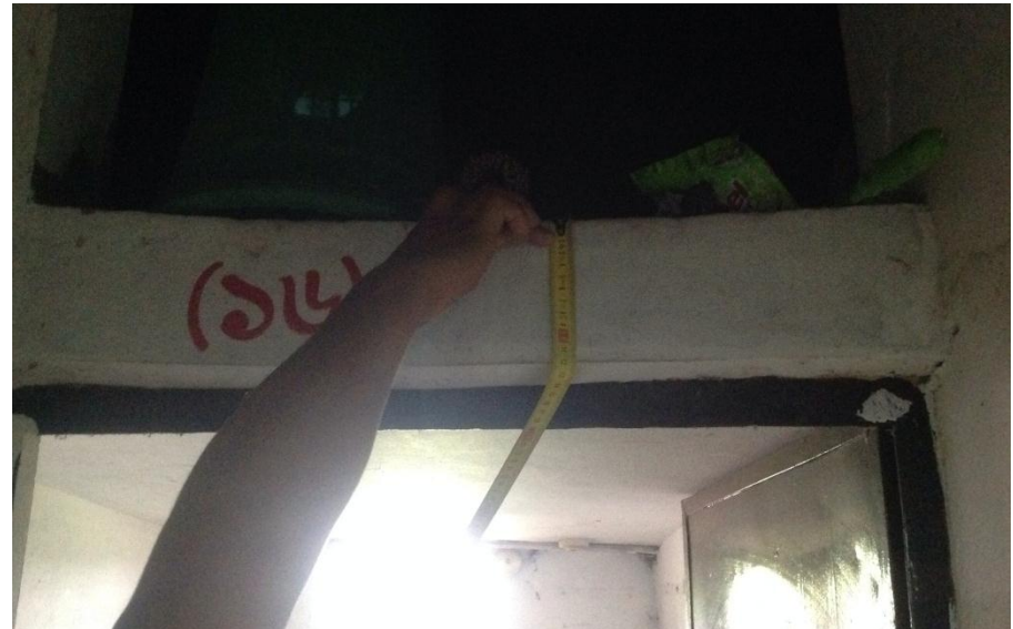
120mm Suspended slab to 1 st Floor Toilet
