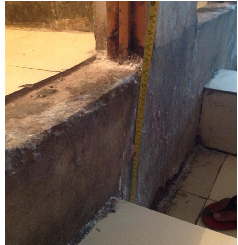
500mm Toilet Plinth to 3 rd Floor
