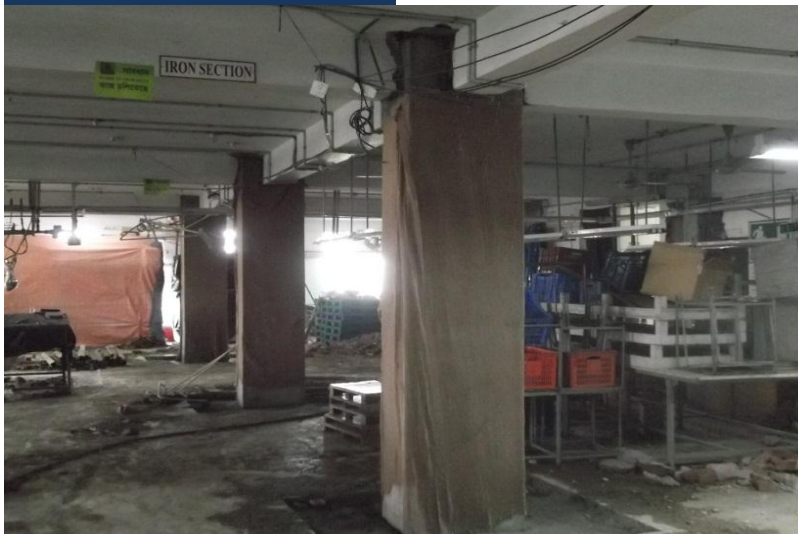
Column strengthening works at Ground Floor
