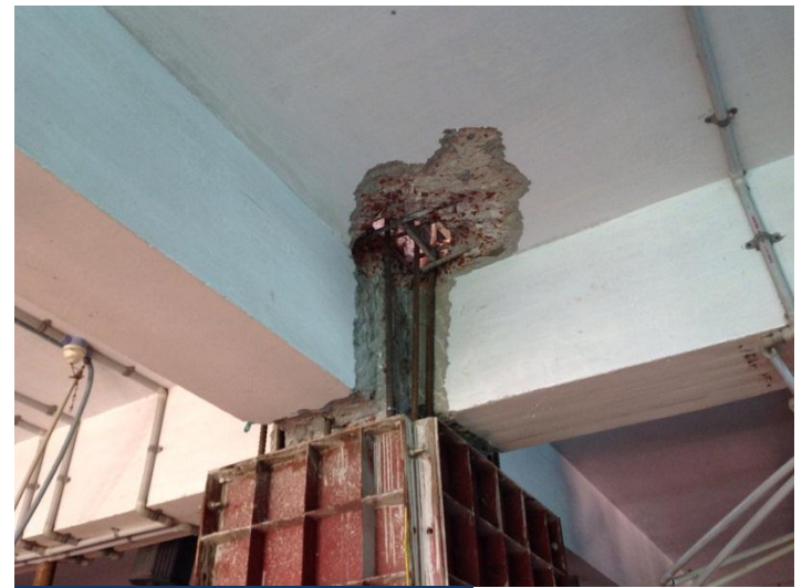
First floor soffit level
