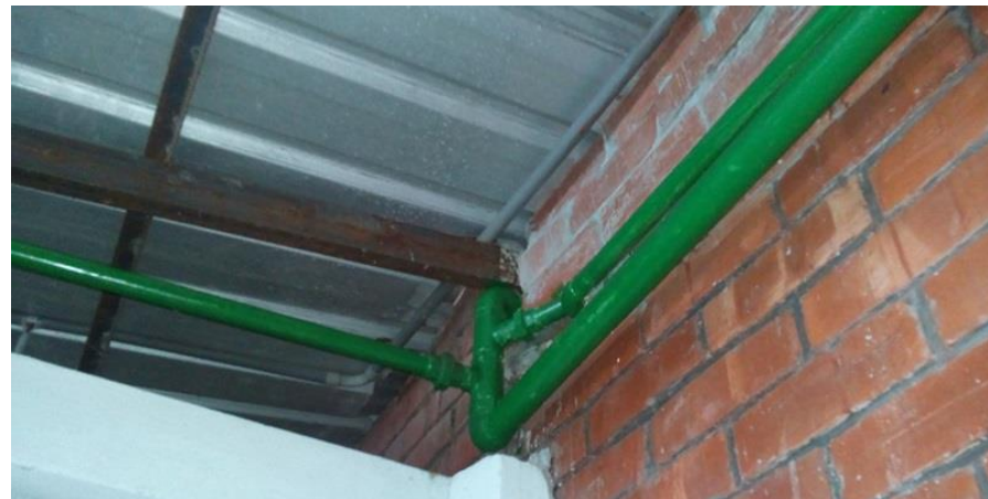
Joint with production shed
