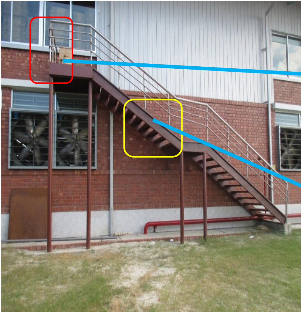
Non-engineered steel stair at north
