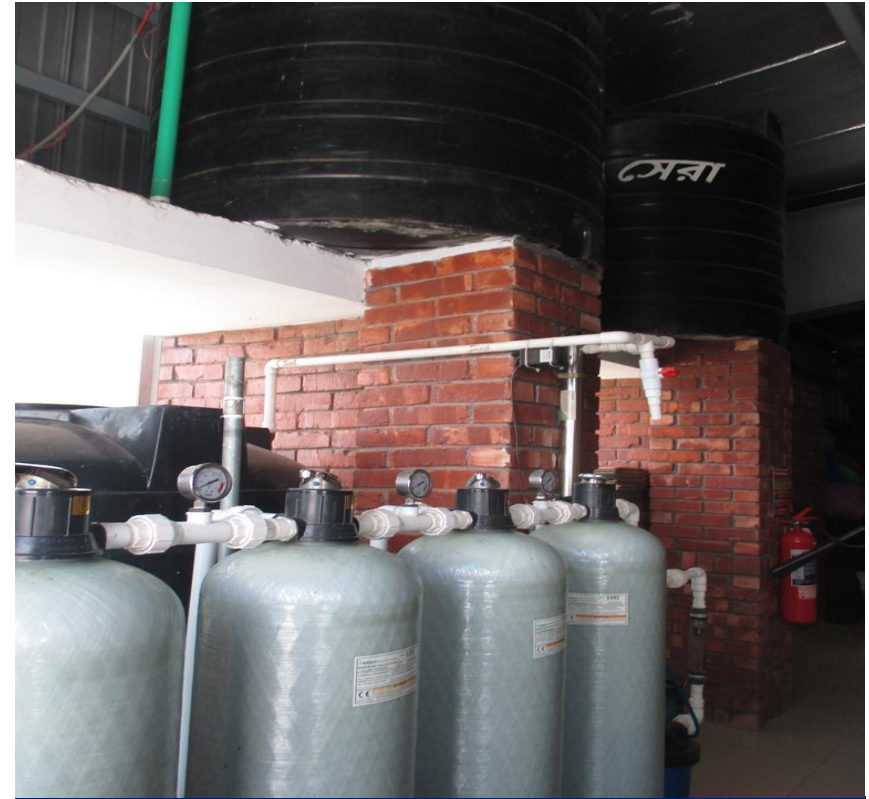
3 nos of plastic water tank found at north-west corner on mezzanine floor .
