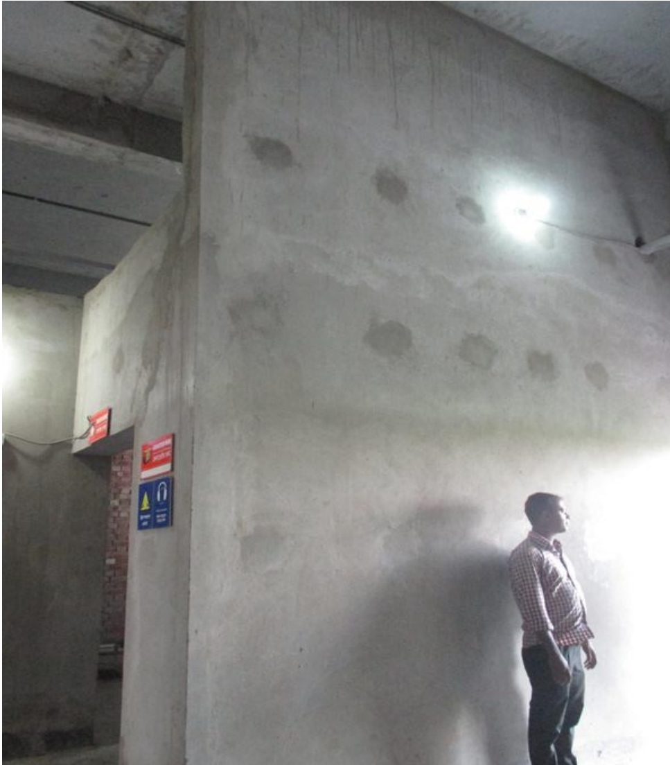
Unsupported 10" Brick wall observed
