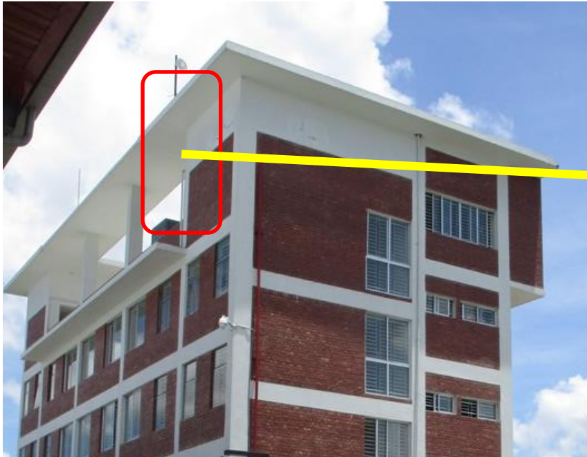
RC slab at roof
