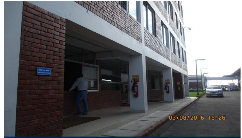
Column size measured 425X300 & 4x3 nos of rebar found
