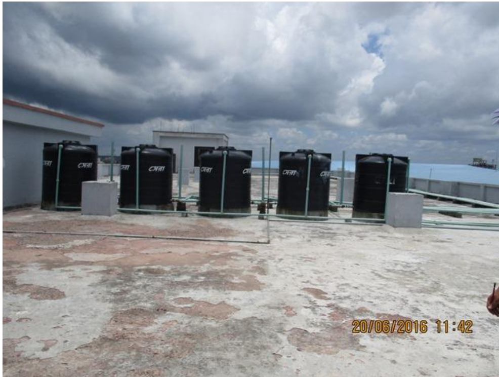
Damaged water proofing material at roof.
