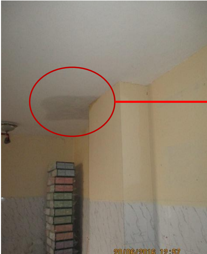
Dampness observed at GF floor slab under toilet area.
