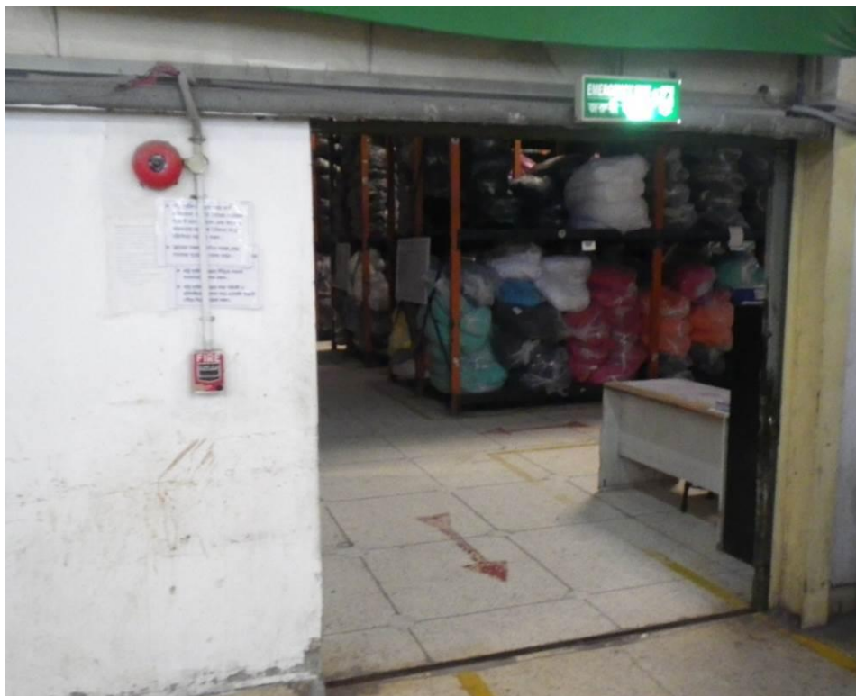
Photo 14 – Egress through storage warehouse (Dyeing-1)
