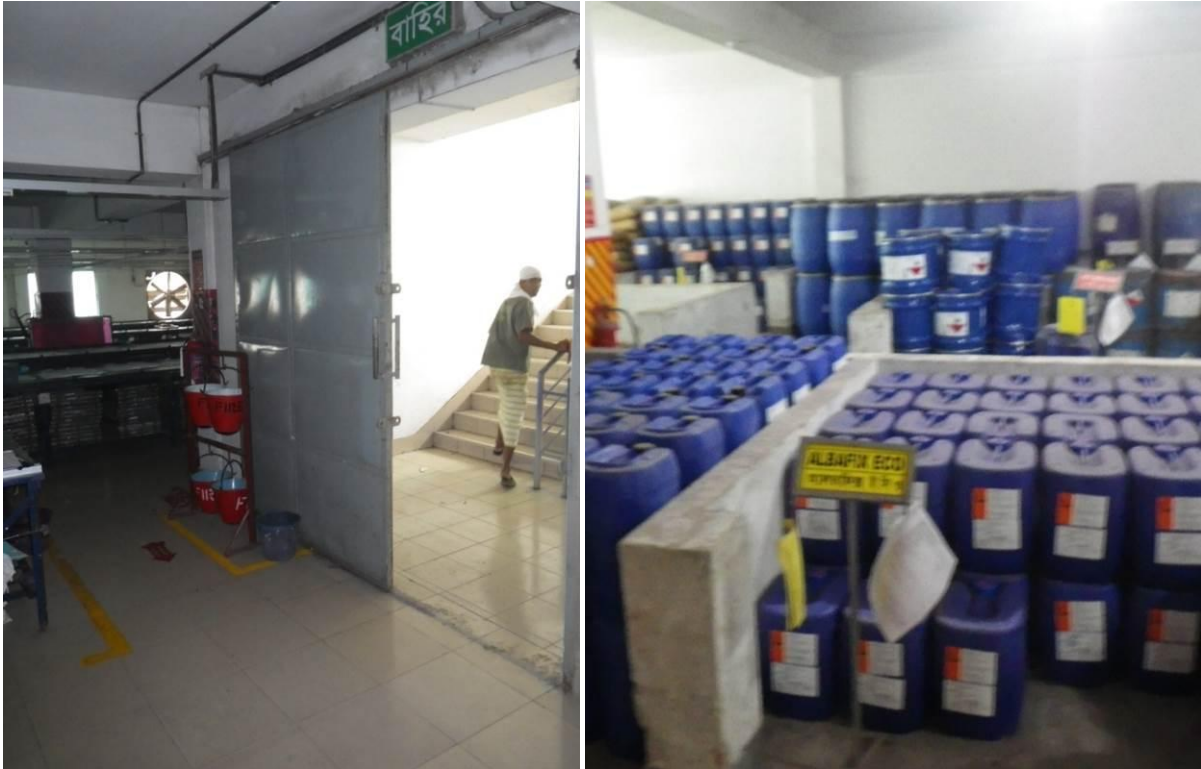
Photo 13 – Chemical storage, not separated from exit stair serving production floor (GMT-2)
