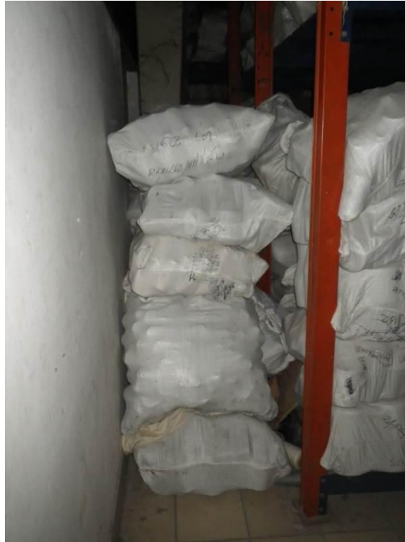
Photo 19 – Storage creating dead-end aisle in warehouse (Knitting)
