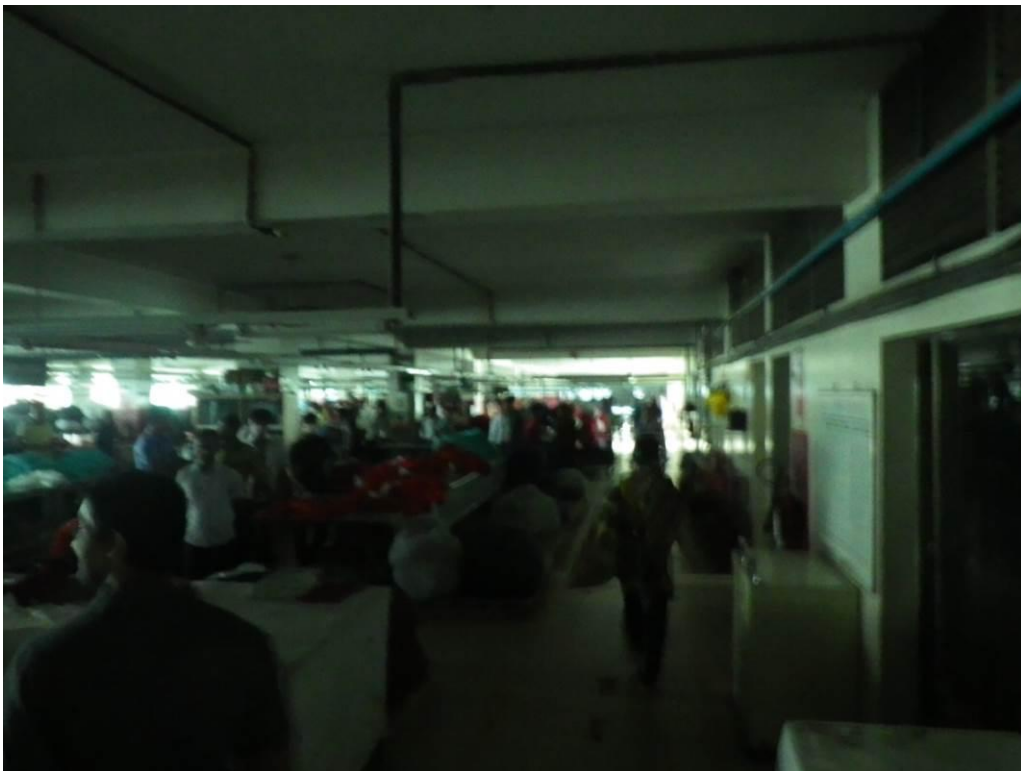
Photo 12 – Production floor operating without normal/emergency lighting (GMT-2)
