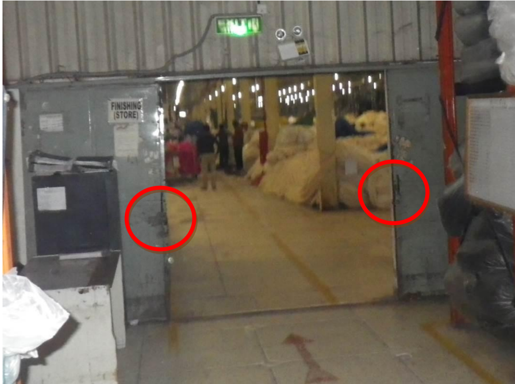
Photo 15 – Sliding egress door with locking features (Dyeing-1)
