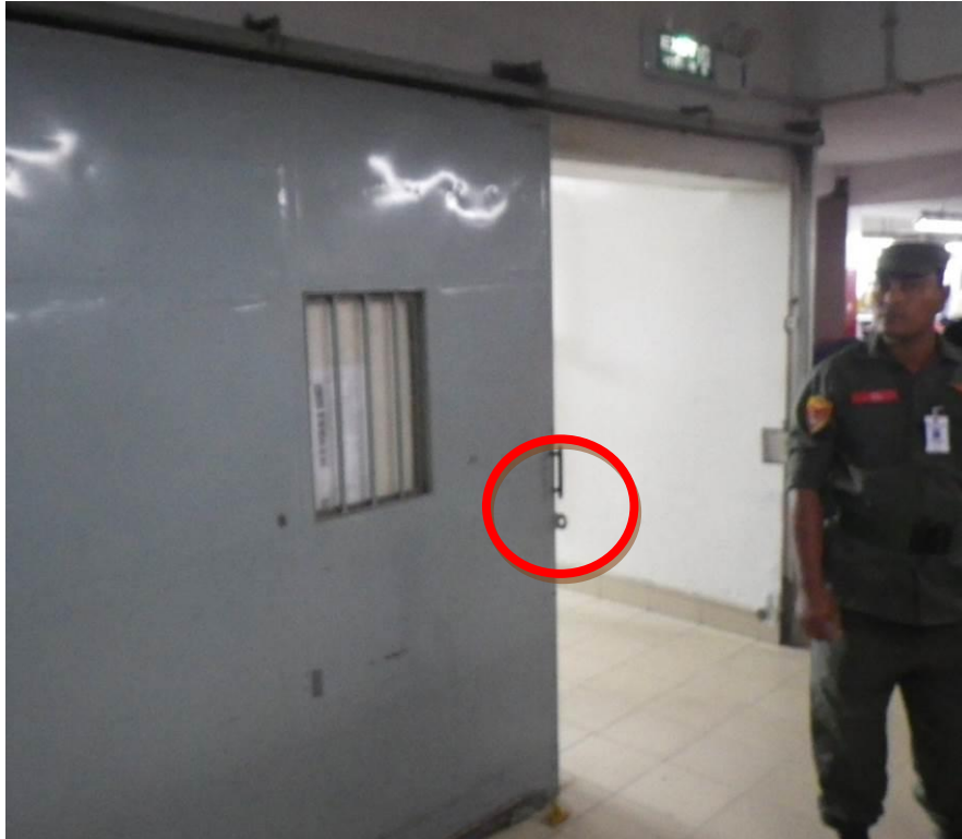
Photo 9 – Non-rated, sliding exit stair door with locking features (GMT-2)
