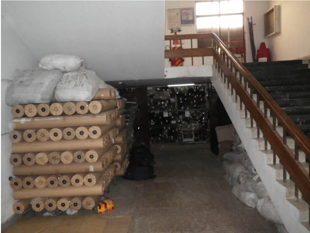
Photo 15 – Storage located in exit stair
