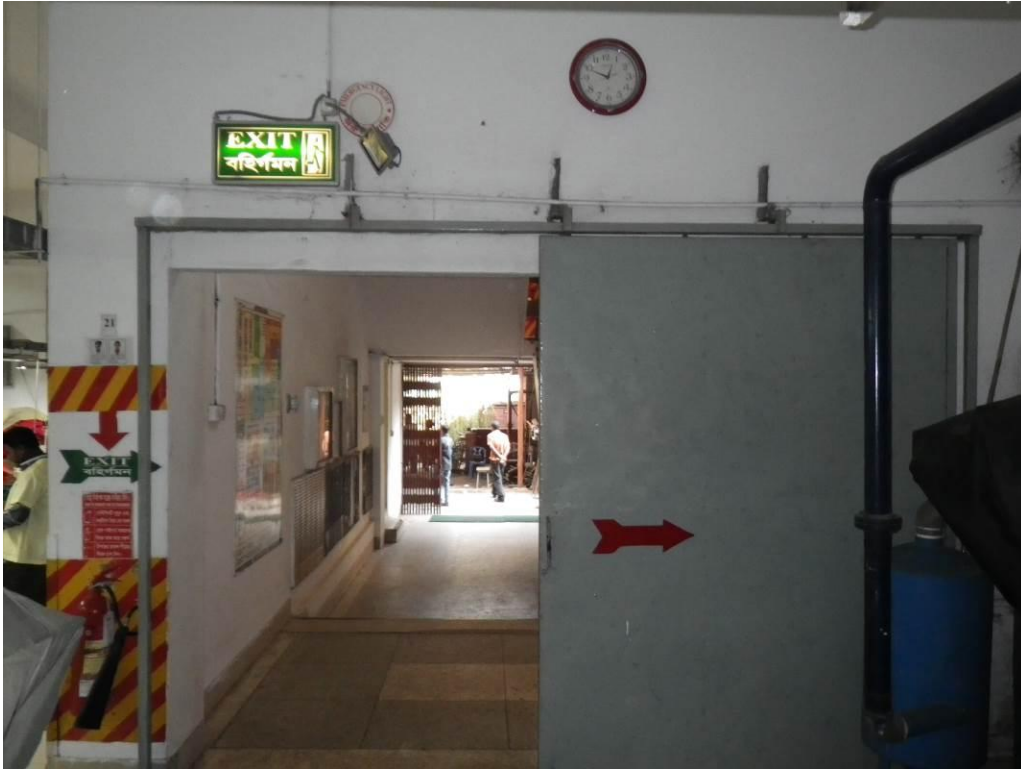
Photo 1 – Exit stair open to production area (typical)
