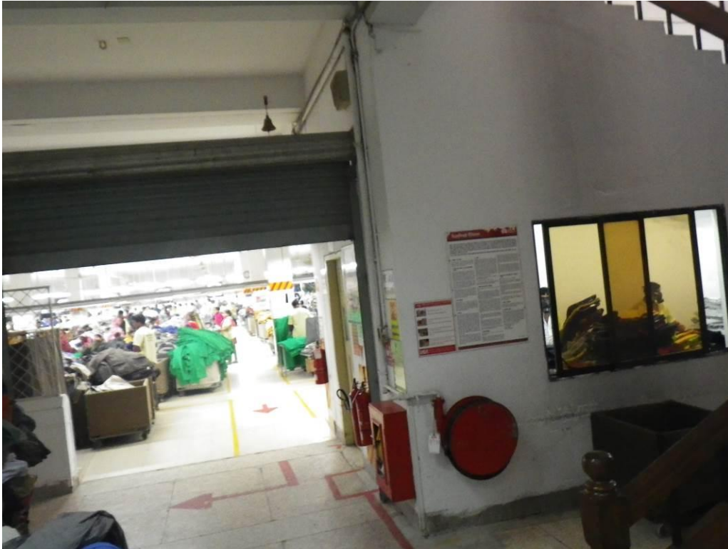
Photo 3 – Exit stair open to production floor with spot cleaning room under the stair
