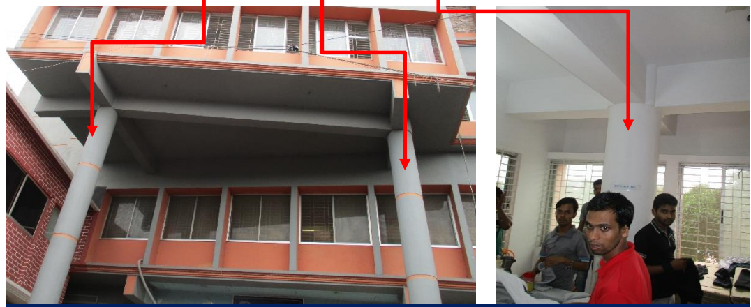
Circular columns in 1 st and 2 nd floor
