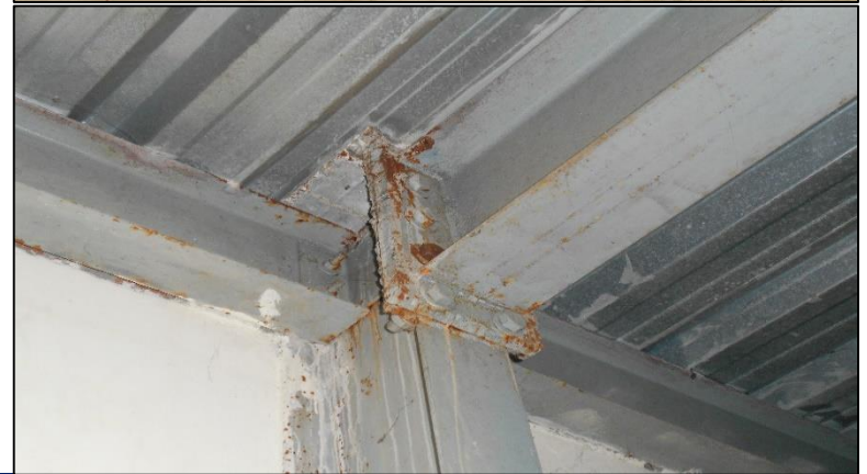
Lack of engineered connection between columns & beams and loose bolts at column base
