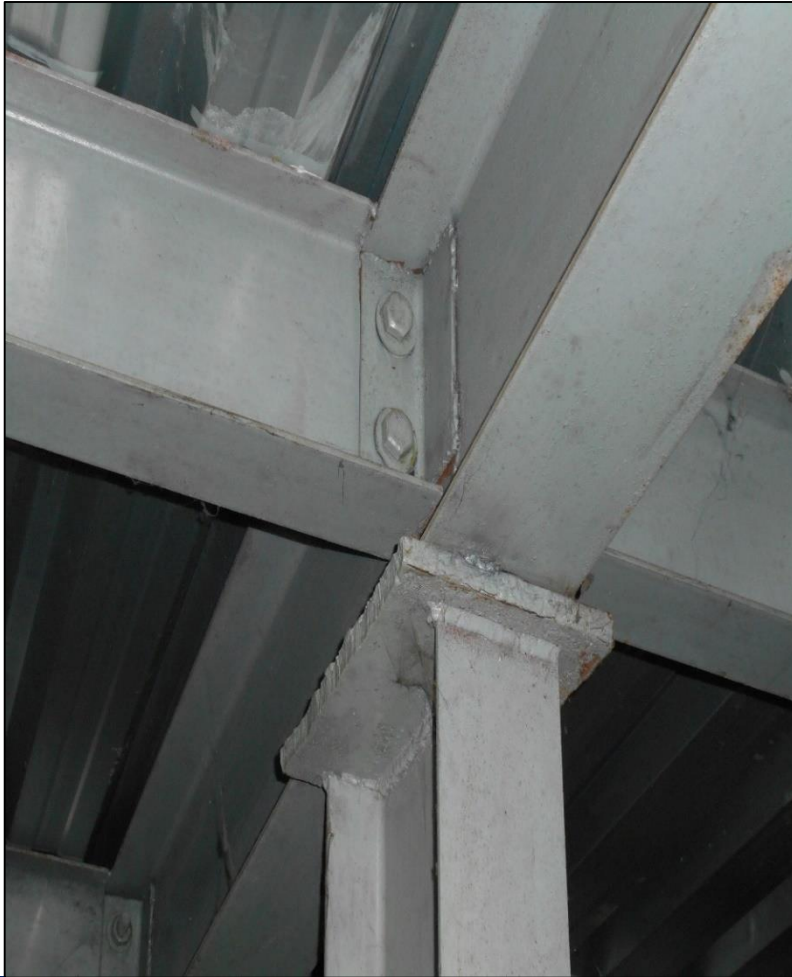
Lack of engineered connection between columns & beams and loose bolts at column base
