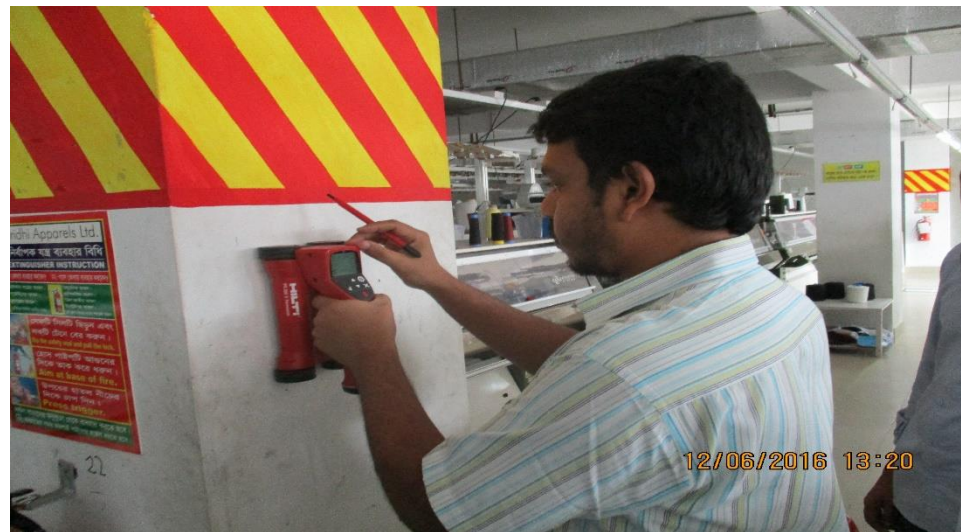
Column rebar checking
