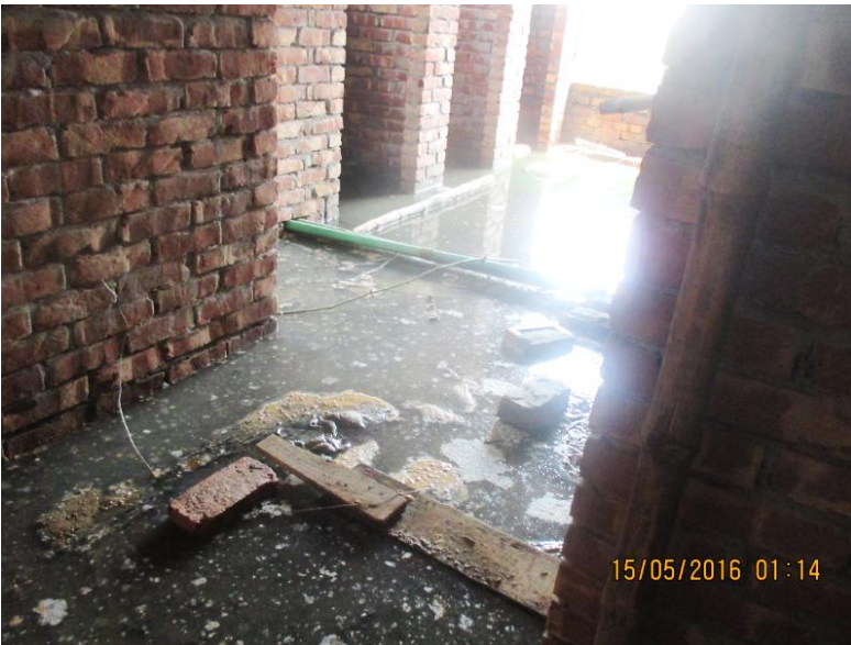
4 th Floor Toilet Area- Factory Building
