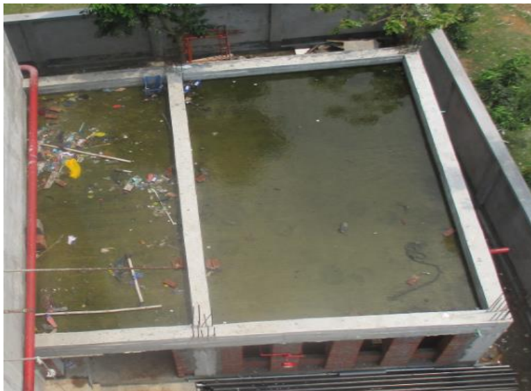
Roof- Pump House
