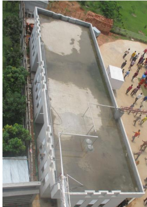
Roof- Utility Building
