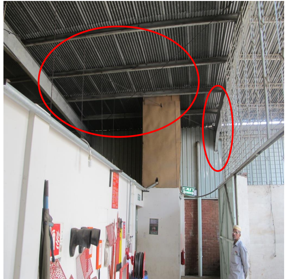
Portal rafters in Storage annex are a continuation of portals in Main Production shed, 6 portals to form a 5-bay wide storage shed
