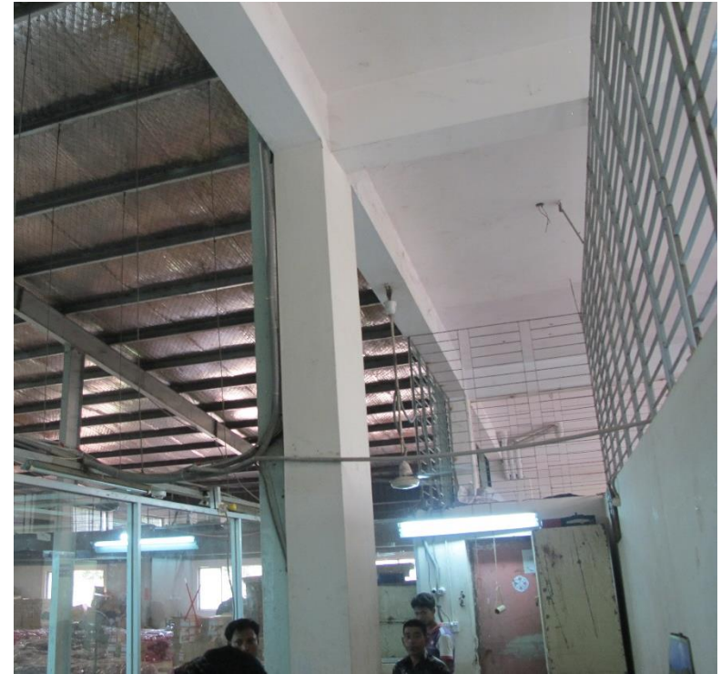
Typical beam and slab structure looking at 1 st Floor from Ground Fl
