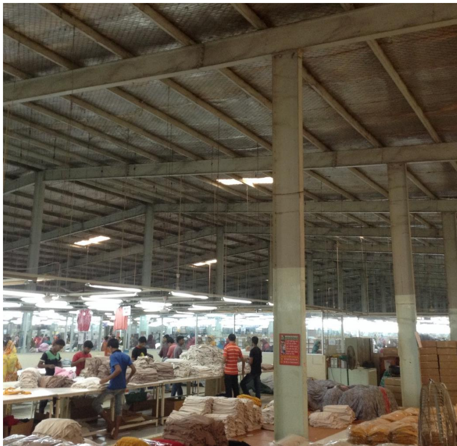
Typical Beam Column portal frame
