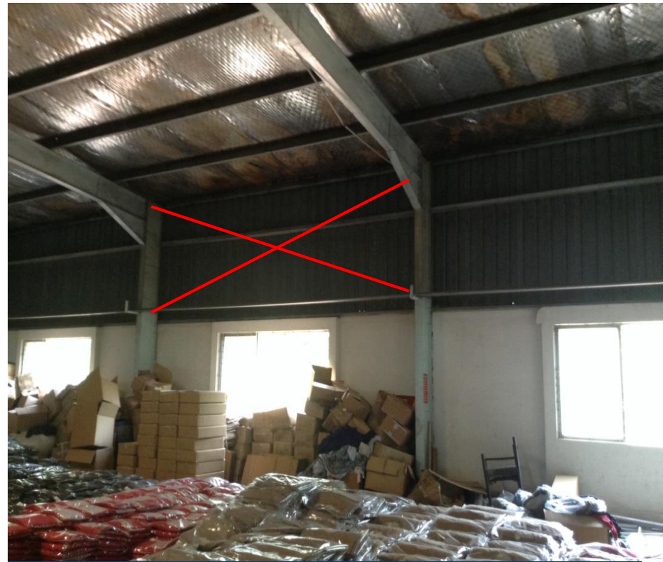
No cross bracing from eaves of the steel portals to the top of the brick wall The steel column cleats welded onto them and built into the top of the 2.65m brick wall to provide lateral stability at this level.
