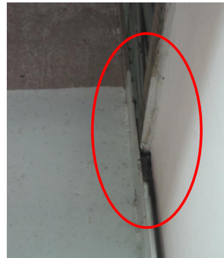
Cleat welded to Steel Column and built into the brick wall
