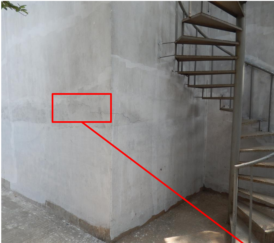
At annexe building (Utility building at ground floor)
