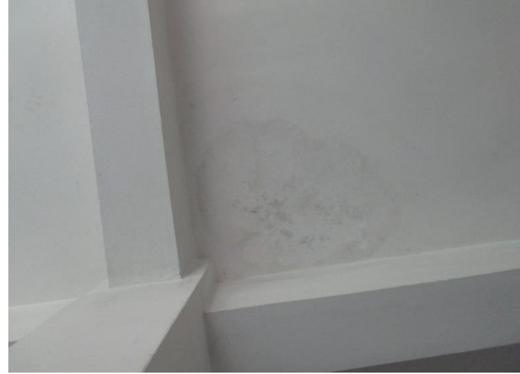
Water ingress in slab due to standing water
