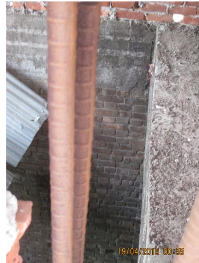
Corrosion in exposed rebar
