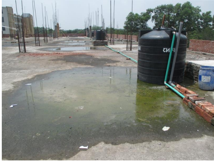
Water ingress in slab due to standing water
