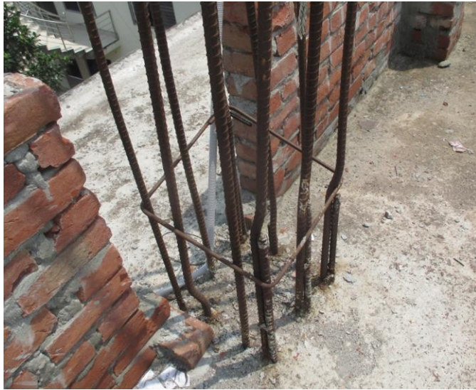
Corrosion in exposed rebar
