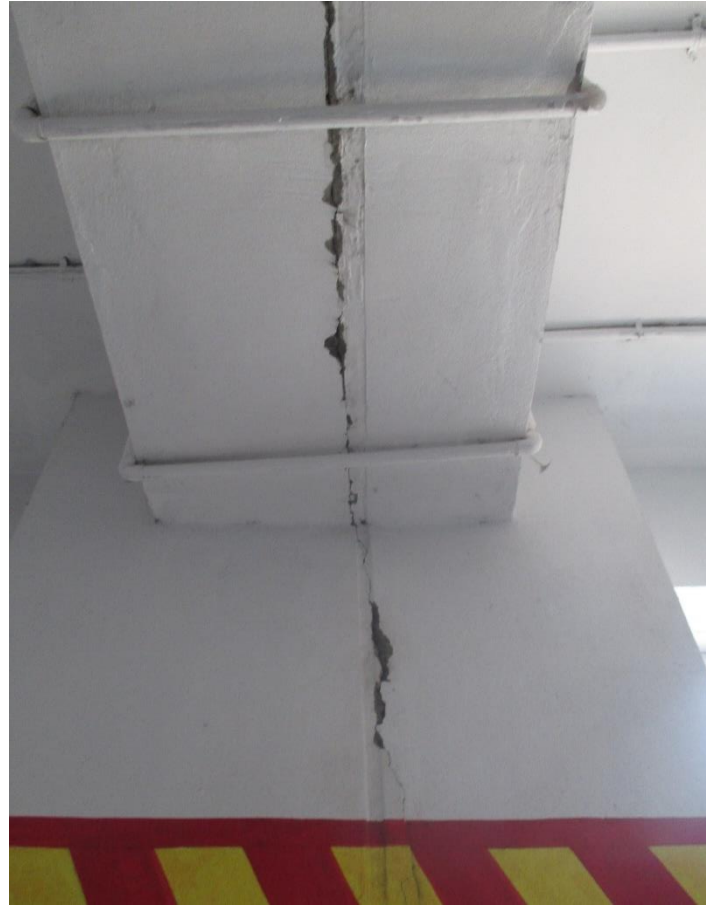
Expansion joint between two columns
