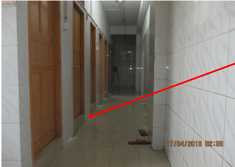
Toilet build up
