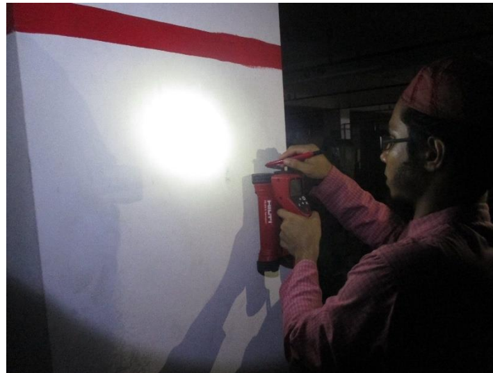
Column rebar checking
