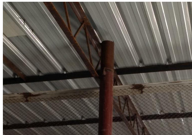
Non-engineered connection
