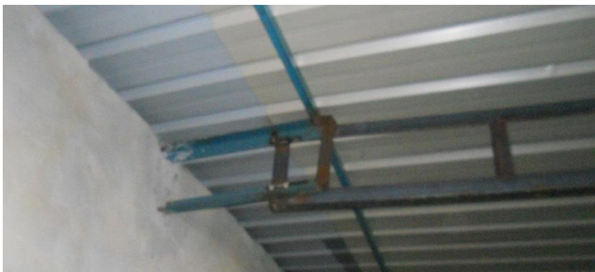
Non-engineered connection
