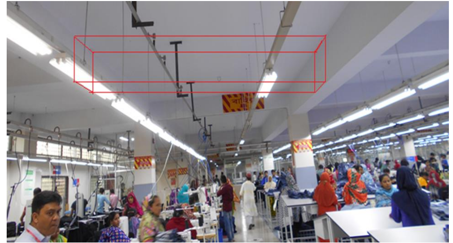
Discontinued beam in every floor on several grid
