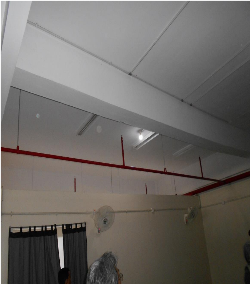
Deflected beam with crack observed in 5 th Floor of the building.
