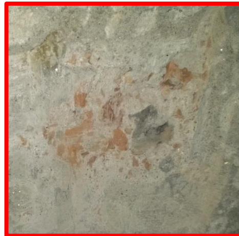
Tested column at lower floors - Brick aggregate observed.
