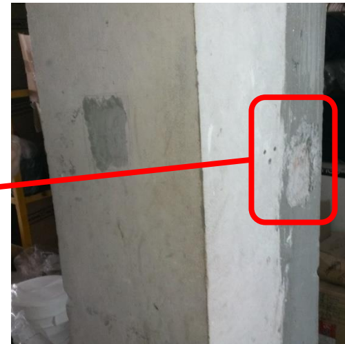
Tested column at lower floors - Brick aggregate observed.
