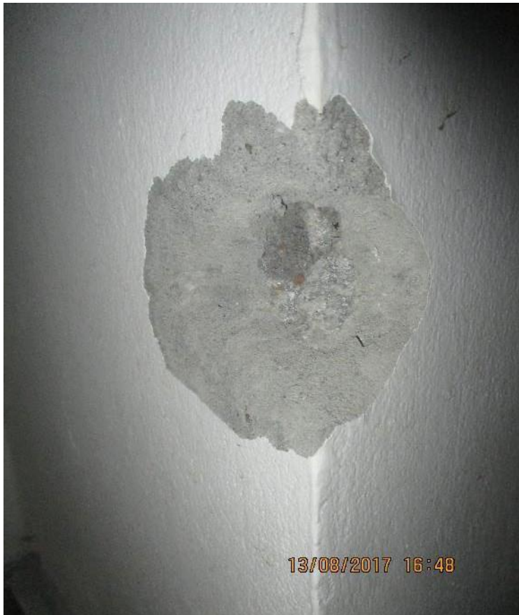
Checking aggregate of column (Stone Chips)
