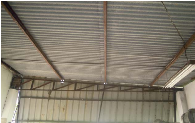
Concrete frame + light steel roof - ETP
