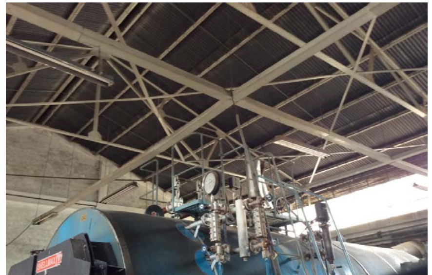
Steel roof supported on steel trusses: Building 3
