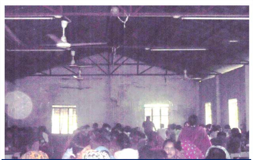
Light steel trusses on masonry walls - Dining
