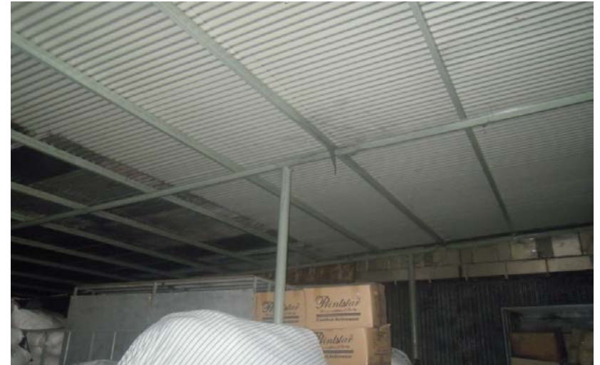
Light Steel Structure - storage
