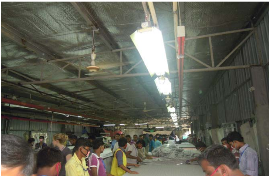
Steel truss supported on steel column: Building 4
