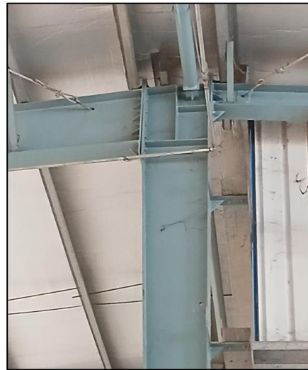
Flange brace missing adjacent to ridge
