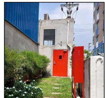
Transformer Control Room
