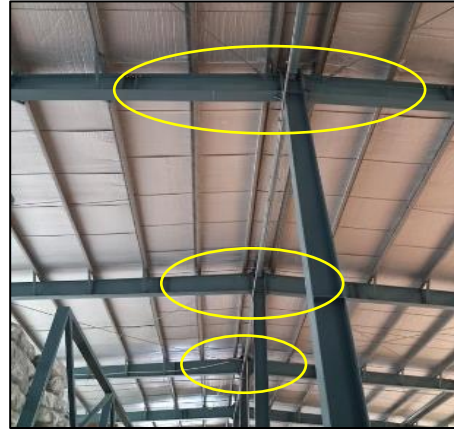
Flange brace missing adjacent to ridge
