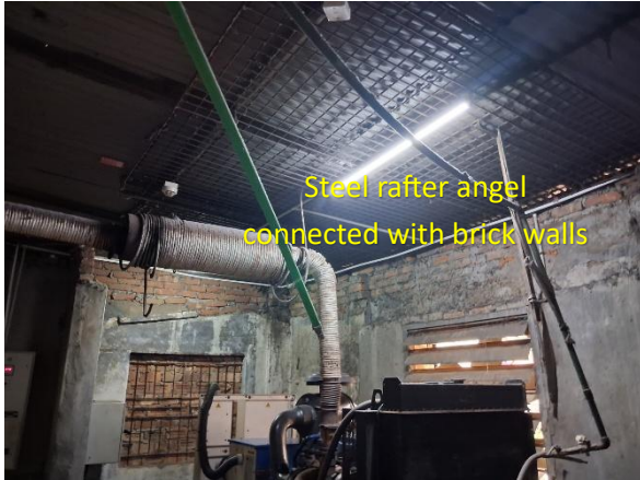
CMB Generator shed
